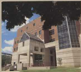
The UTK Science and Engineering facility, the largest campus building designed exclusively for research, was dedicated. The structure is a research laboratory of "building behavior": sensors in the foundation monitor settling and wind load.
