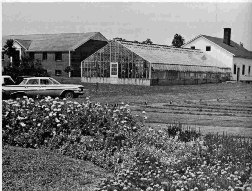
Office building (left), and greenhouse and headhouse (right), at the Tobacco Experiment Station, Greeneville. In the foreground are experimental plantings of flower borders and turfgrasses.
