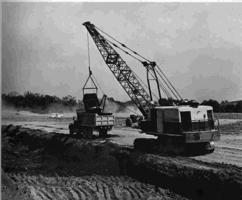
Phosphate mining in Middle Tennessee. The soil over the phosphate is removed and deposited on mined land to the left. The phosphate is loaded into trucks for transport to the plant. Reclamation of the mined land for crop production is under study by U-T.
