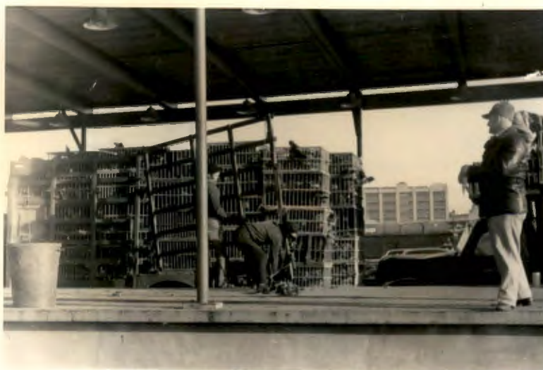
Figure 111. Replacing truck sidings after inspection, New York Live Poultry Terminal, November 1942.
