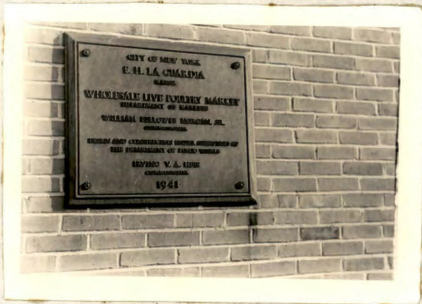
Figure 98. Dedication plaque on office building, New York Live Poultry Terminal, November 1942
