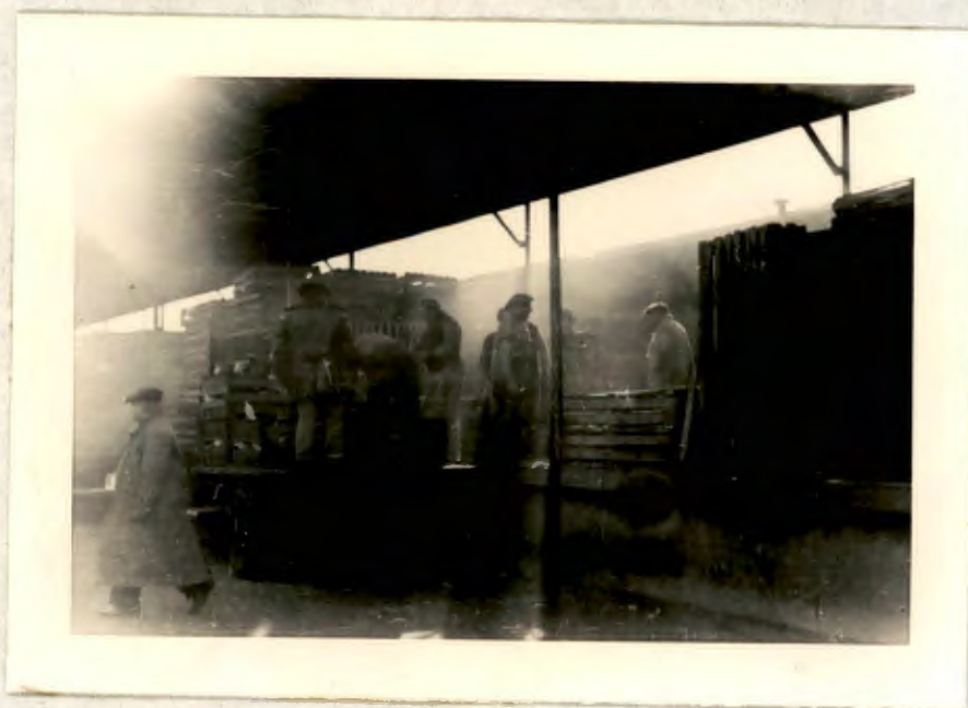
Figure 114. Loading buyers' trucks from car unloading platforms, New York Live Poultry Terminal, November 1942.
