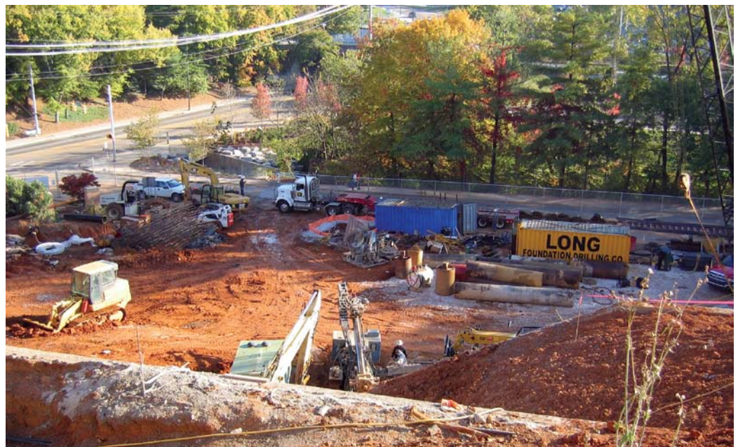
Construction has begun on the new Min H. Kao Electrical Engineering and Computer Science Building
