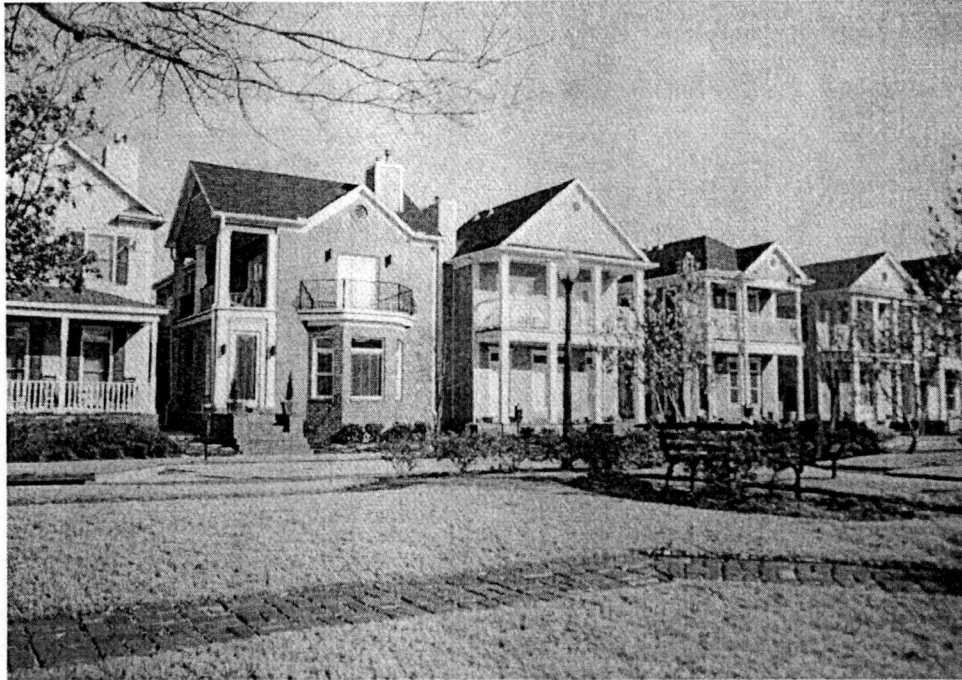
Figure 4-11. Houses along Boulevard, South Bluffs
