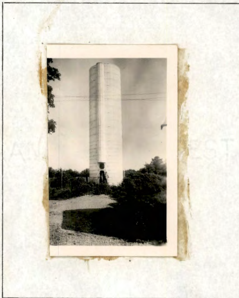
Figure 6. A 12x45 Foot Roofless Concrete Stave Silo in Good Repair (Farm of D. D. Cantrell, Rutherford County, Tennessee, 1948 - Capacity 120 tons)
