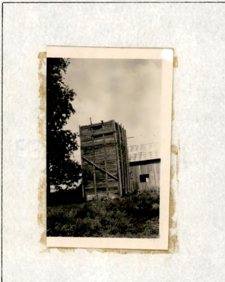
Figure 2. A 10x12x20 Foot Home Made Wooden Silo Lined with Used Sheet Tin (in Use on the Farm of Frank Peyton, Rutherford County, Tennessee, 1948 - Capacity 42 tons)
