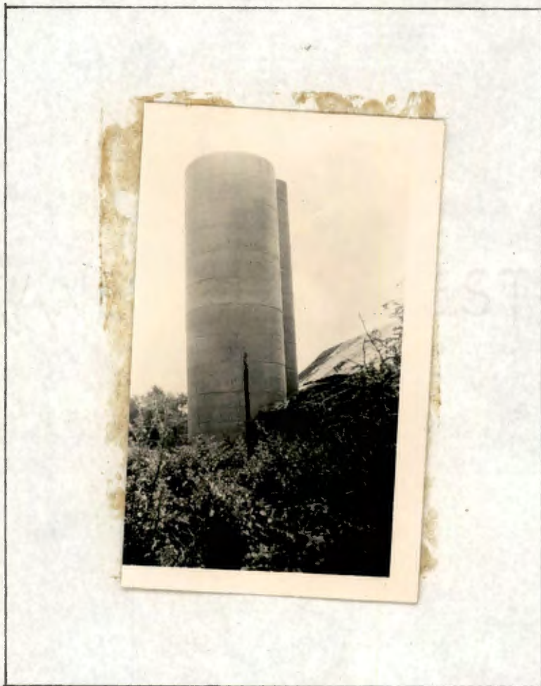
Figure 5. A Usable 10x36 Foot Solid Concrete Silo Which Has Been Abandoned (Rutherford County, Tennessee, 1948)
