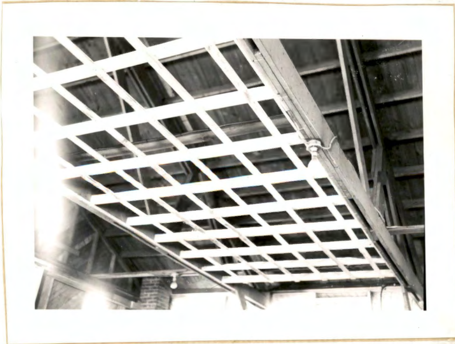
Fig. No. 1 View of the Ceiling Before Panels Were Installed.
