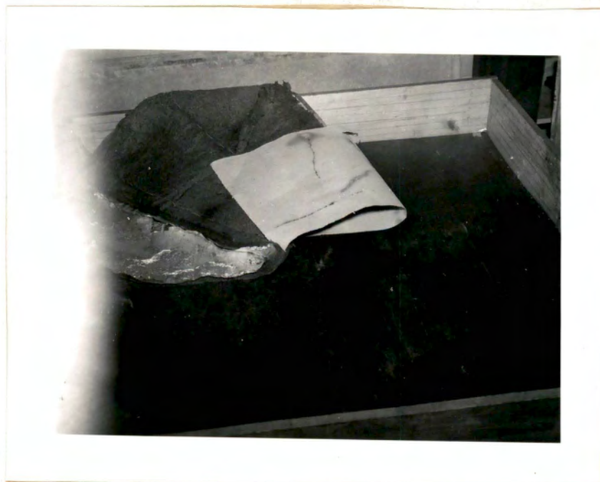
Fig. No. 11 View of Element Cracking.
