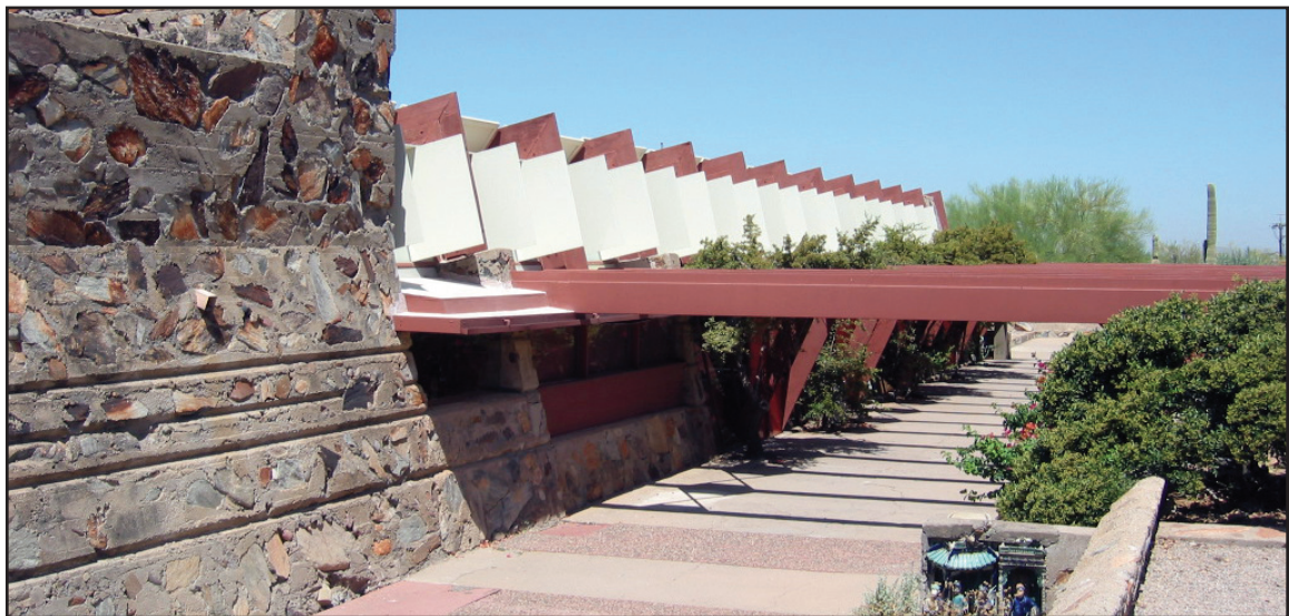
Figure 02.08- Taliesin West Trellised Walk (Photo by author)
