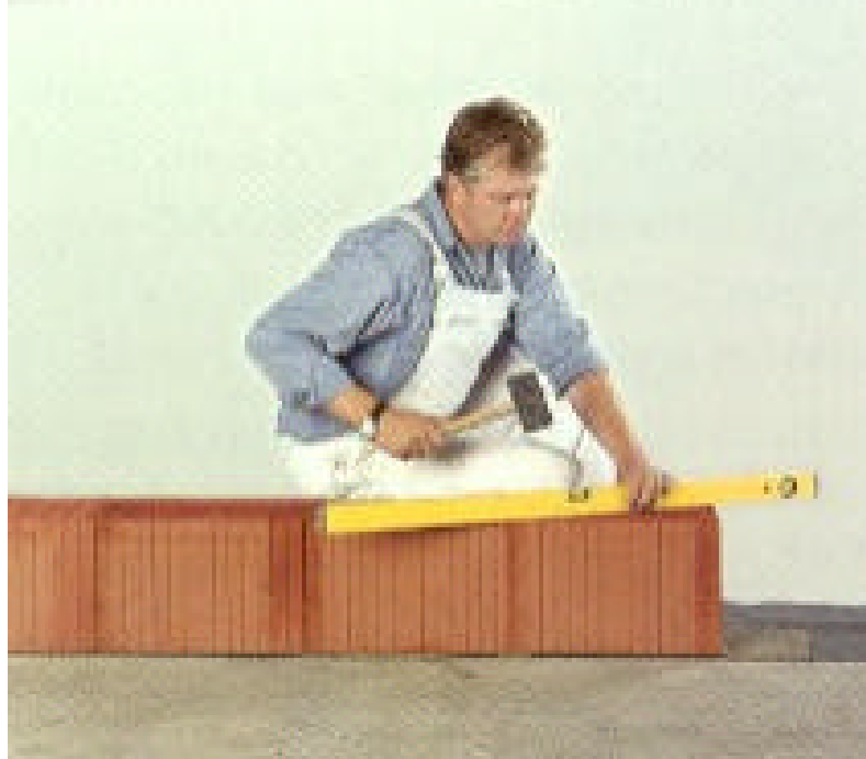
FIGURE 1.2 - First Course Construction
