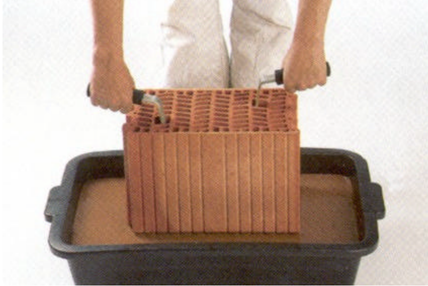
FIGURE 1.4 – Dipping Application of Mortar
