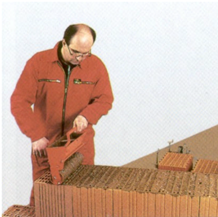
FIGURE 1.3 - Roller Application of Mortar
