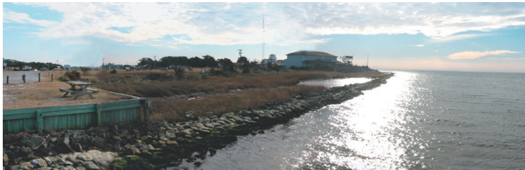
Figure A-22. 1) Southwest View from Public Docks.
