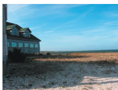
Figure A-4. Looking West.
