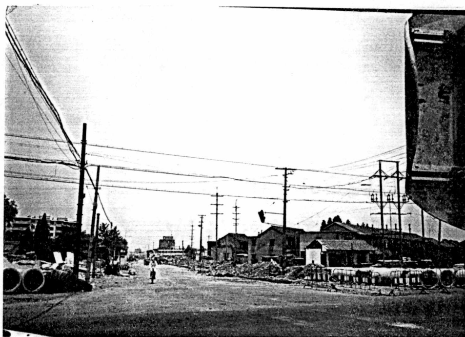
Figure 17: The Construction Sites of Nan Pu Bridge and Yang Gao Road.
