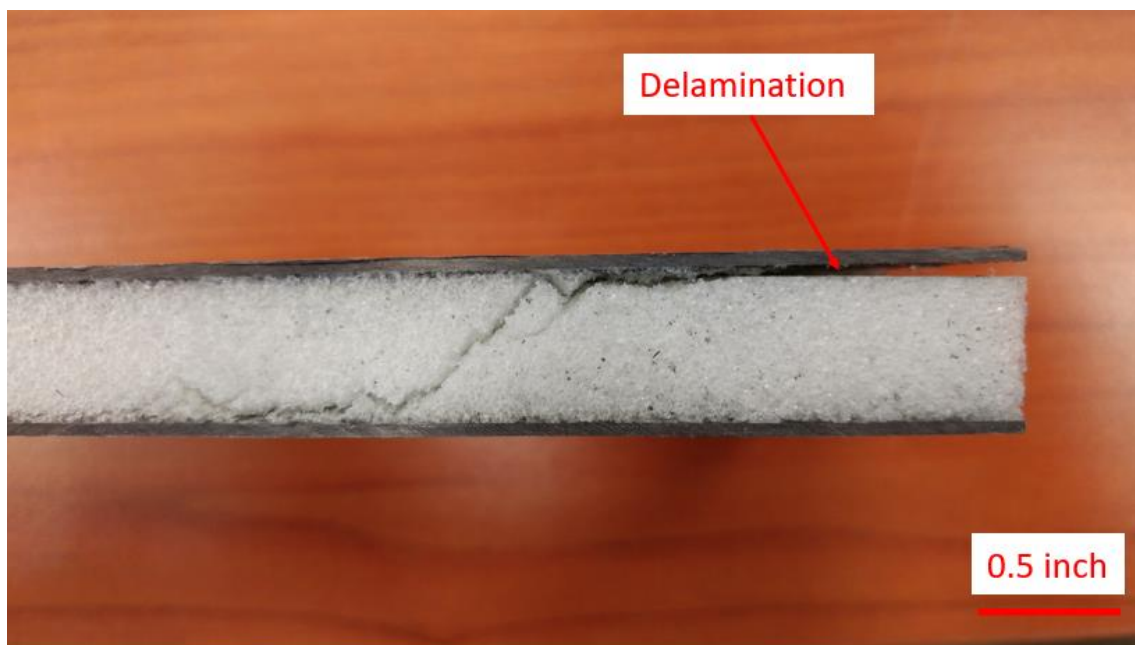
Figure 64 - Delamination due to core shear, visible inspection to compare to non-destructive evaluation
