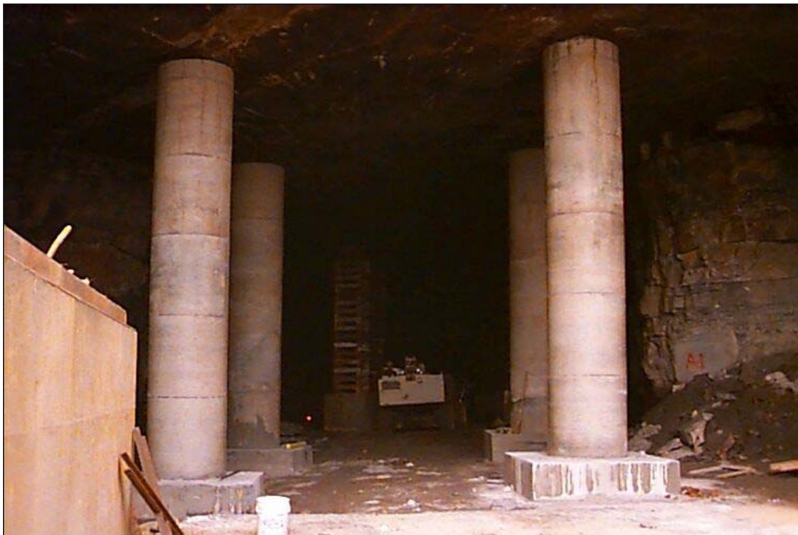
Figure 14. Fort Hartford Mine Superfund Site Cast-In-Place Concrete Columns at “A” Portal
