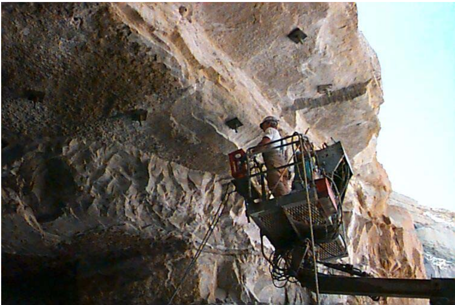
Figure 15. Fort Hartford Mine Superfund Site Installation of Roof Bolts at “A” Portal
