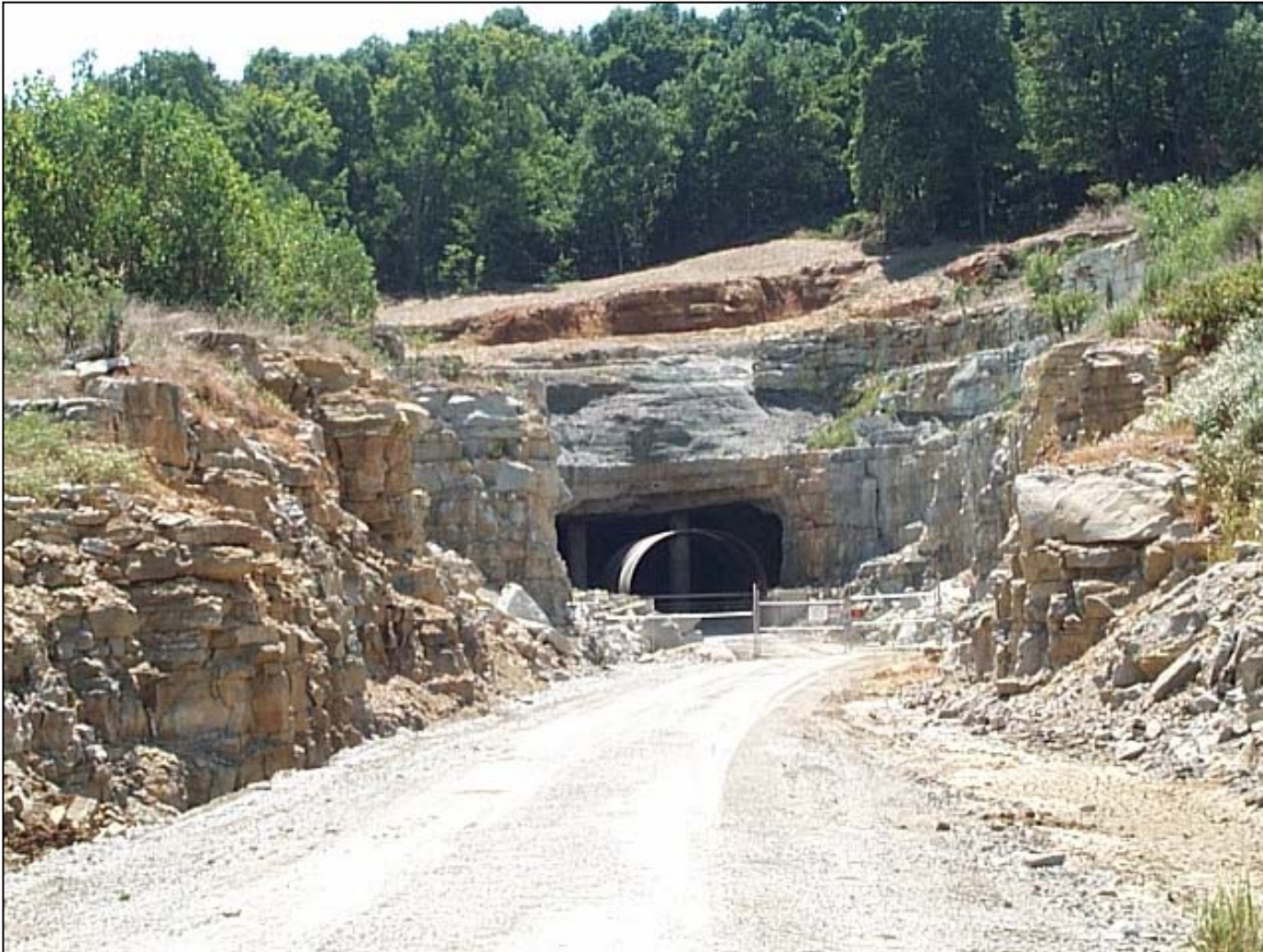
Figure 17. Fort Hartford Mine Superfund Site Repaired Slope at “A” Portal
