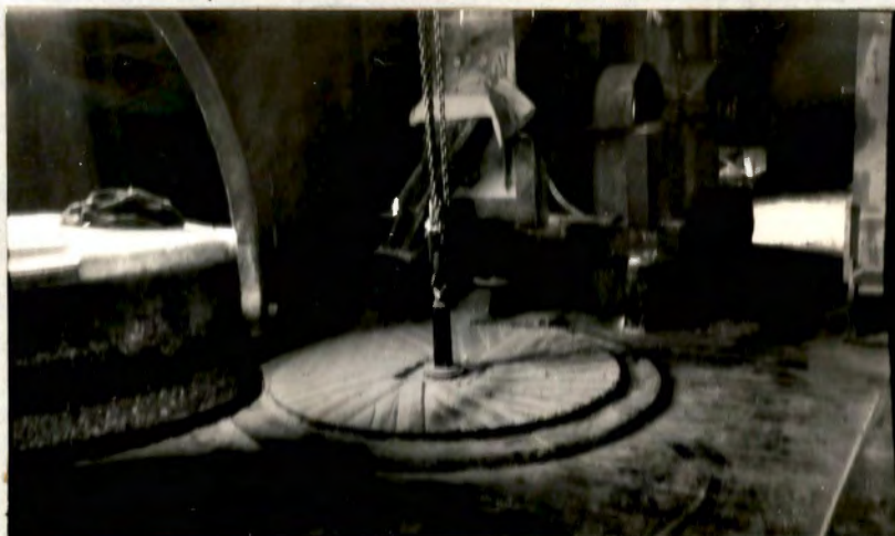
Dismantled burr outfit, smooth stone left, cutting stone in center. Other burr unit is in operation in background
