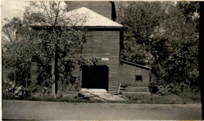
Wheat flour milling unit of 25-barrel capacity; a corn mill unit, capacity 250 bushels daily. Manufactures whole wheat flour and corn meal. Operated by water power. Blount County.
