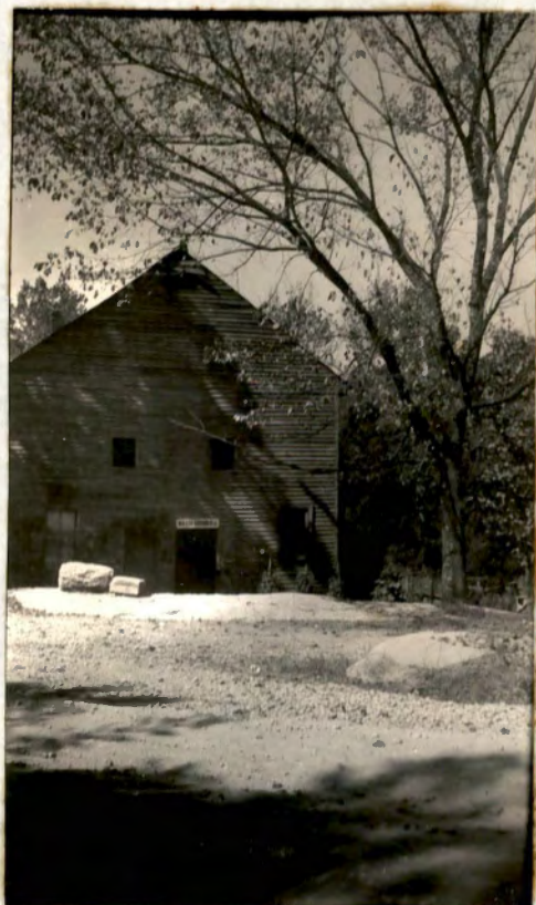
Corn mill. All custom grinding. Milling capacity 1-3 bushels an hour. Operated by water power.
