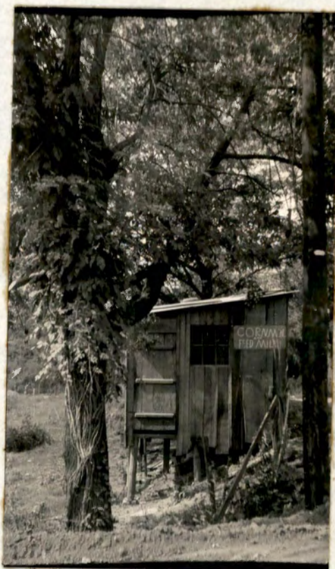
Corn and feed mill. Gas engine furnishes power.
