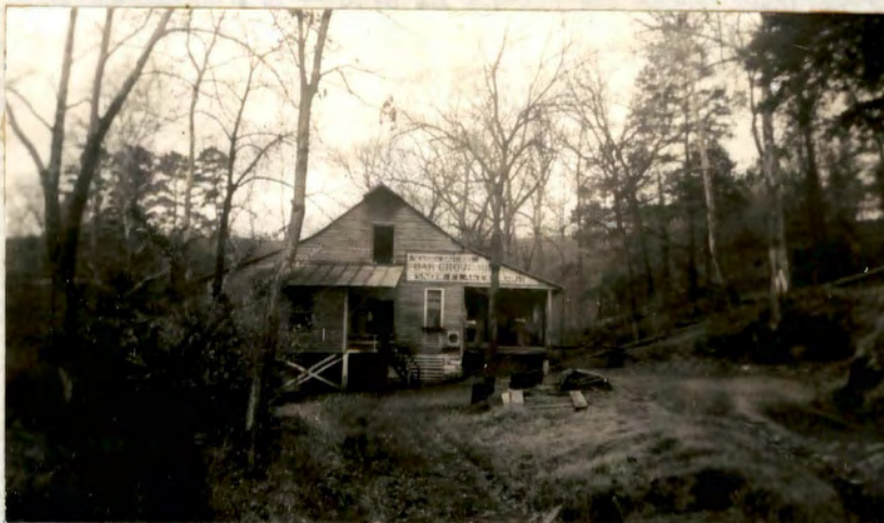
Flour milling unit of 40-barrel capacity; a corn mill unit, capacity 360 bushels daily. Manu- facture Straight Grade flour and corn meal. Operated by water and electricity. Jeffer- son County.
