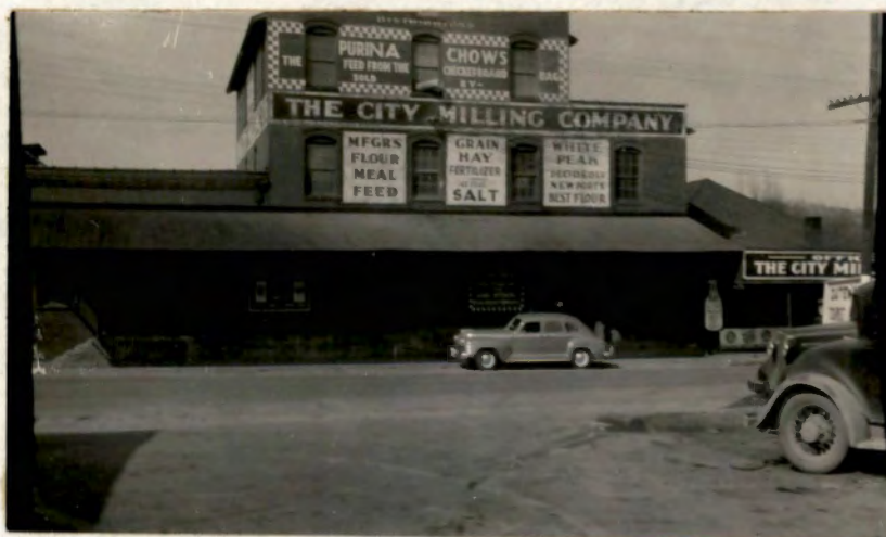
Capacity of mill is 125 barrels of flour, and 500 bushels of corn meal. Power is furnished by electricity. Newport, Cooke County.
