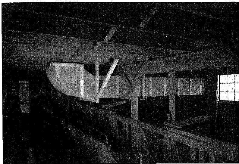
Fig. 6—Delivery duct for conveying air from blower to series of small ducts on floor of hay mow.
