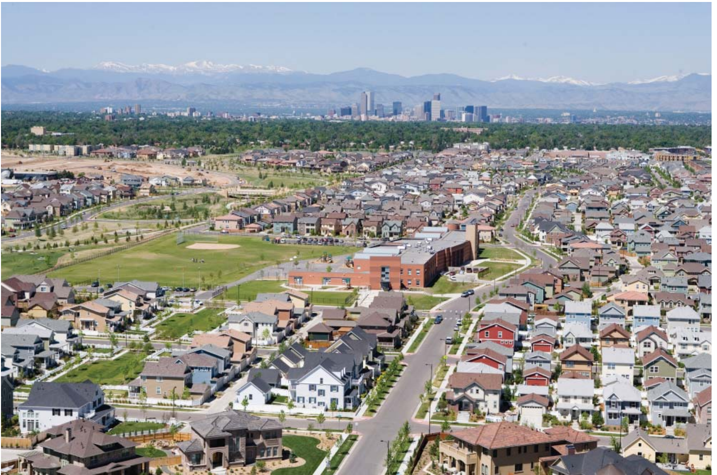
Figure 1: Photograph of Stapleton (n.d.). Note: copyright Chris Palmeri
