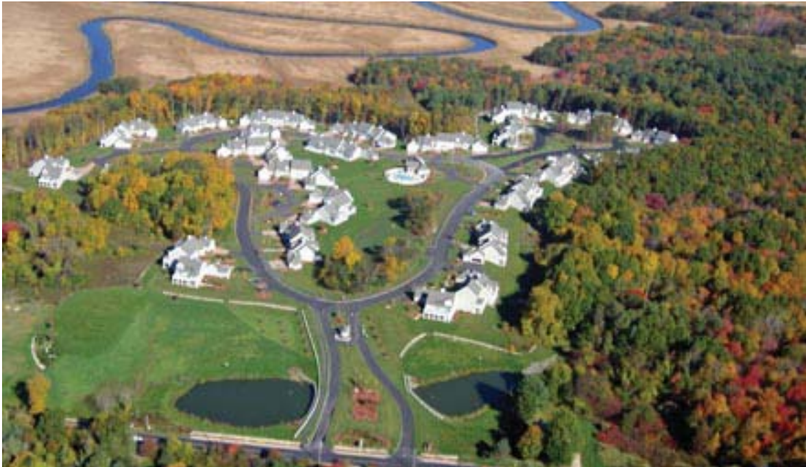
Figure 7: Photograph of Caldwell Farm (n.d.). Note: copyright C.P. Berry Construction
