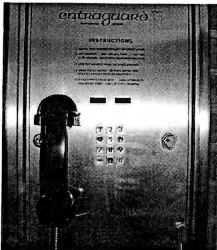
Fig. 50: A phone outside a Center Square Building.
