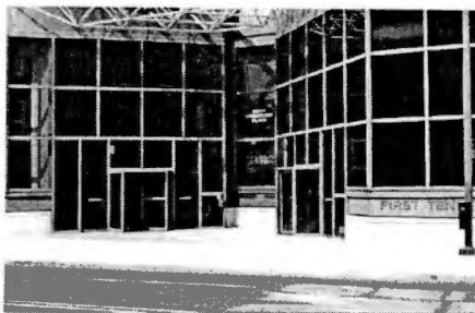
Fig. 46: Entrance to First Tennessee Bank.
