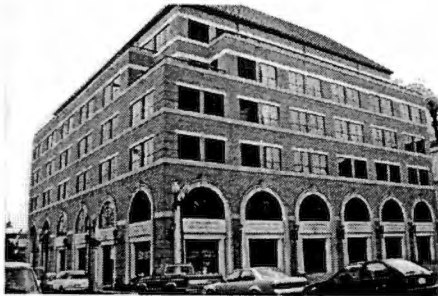
Fig. 48: A facade of a Center Square Building.
