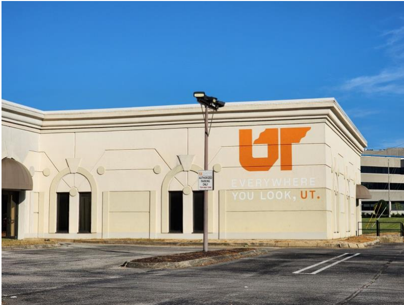
Image: Glazer Building, Oak Ridge, Tennessee
