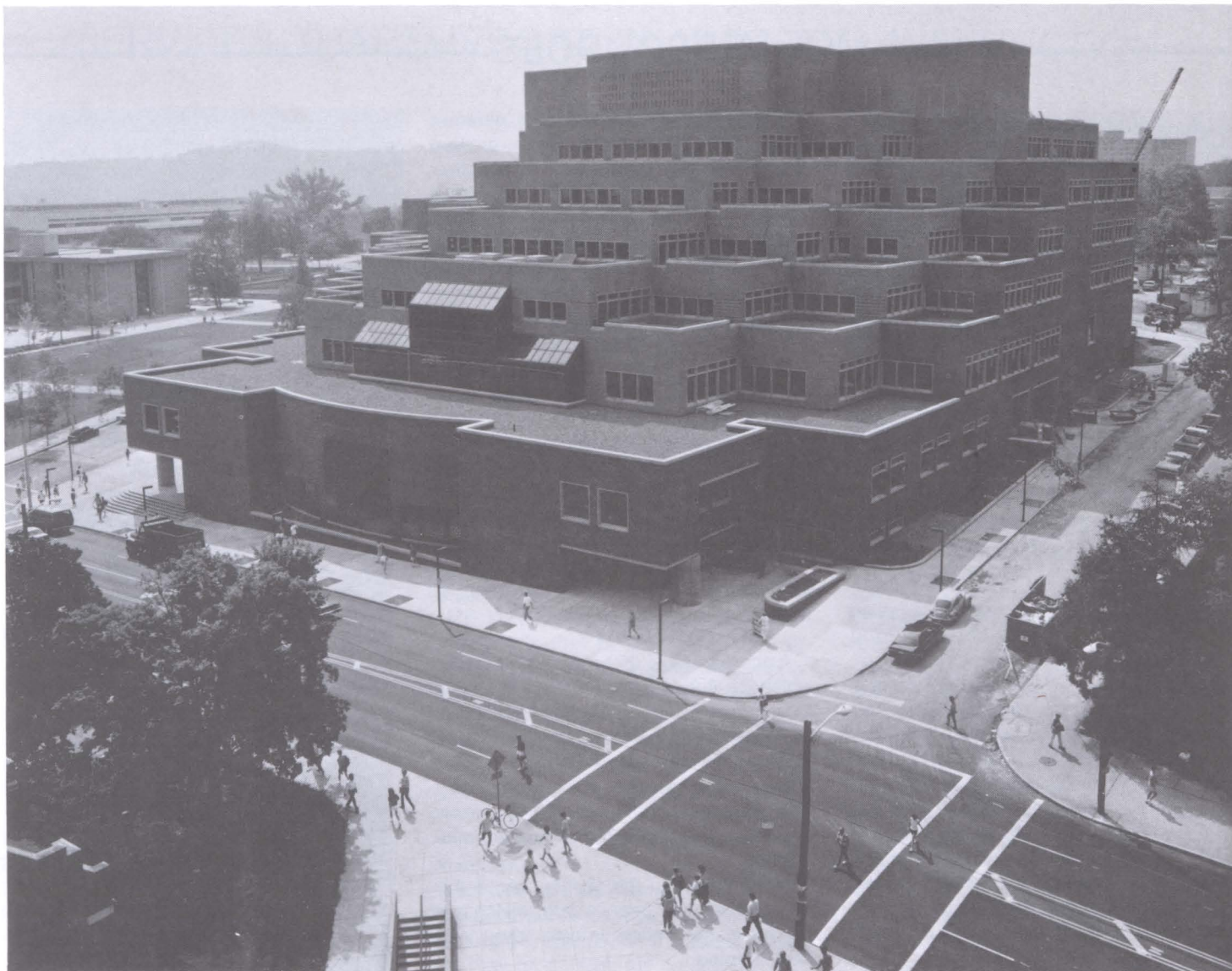
A library in the making—the east face of the new John C. Hodges Central Library, October 1986.
