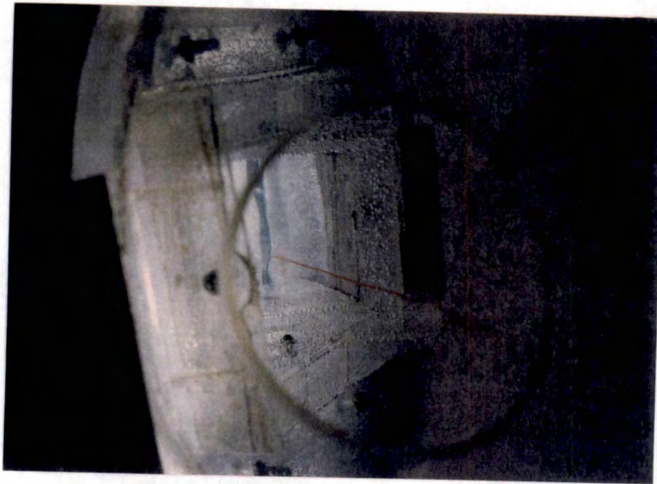
Zone 1, View Upstream into Nozzle Exit
