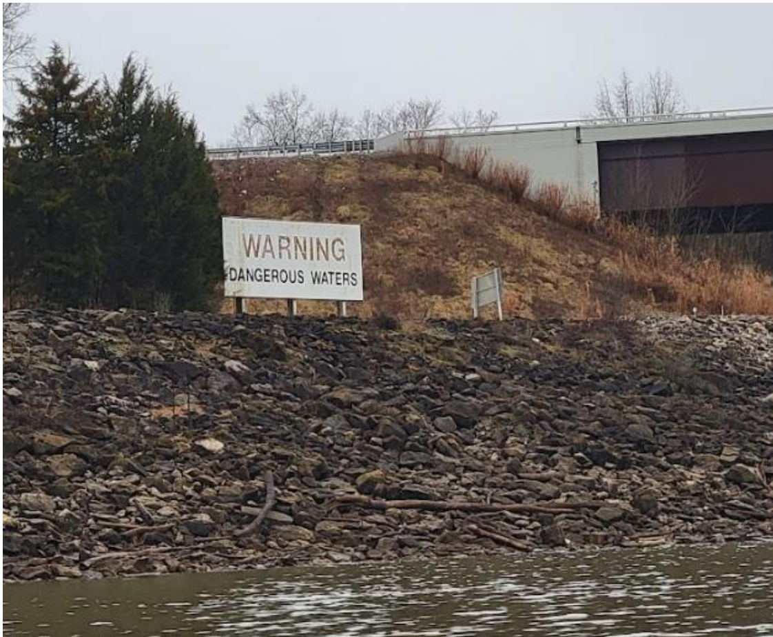
Figure 5. Warning sign along river by Fort Loudoun Dam.
