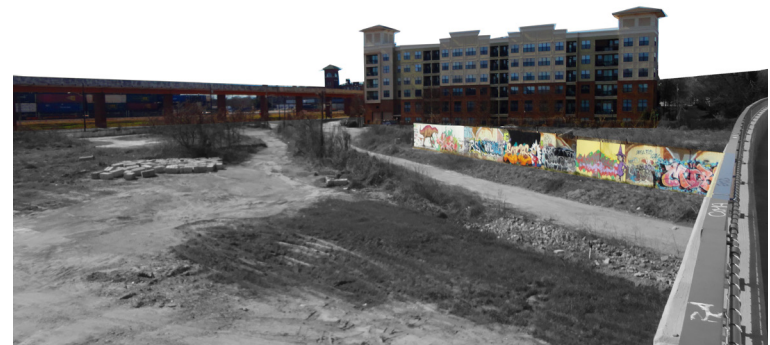
03 | Northeast Approach | Existing Condition
