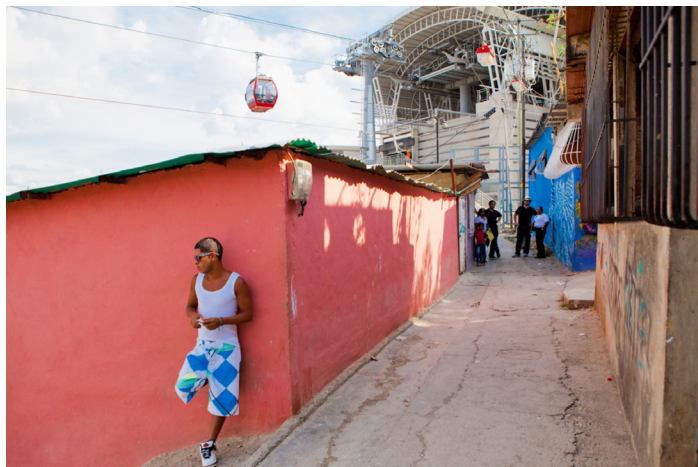
Figure 3.04 Metro Station Entry ( Urban Think Tank )
