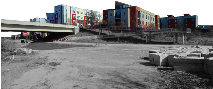
02 | Southwest Approach | Existing Condition
