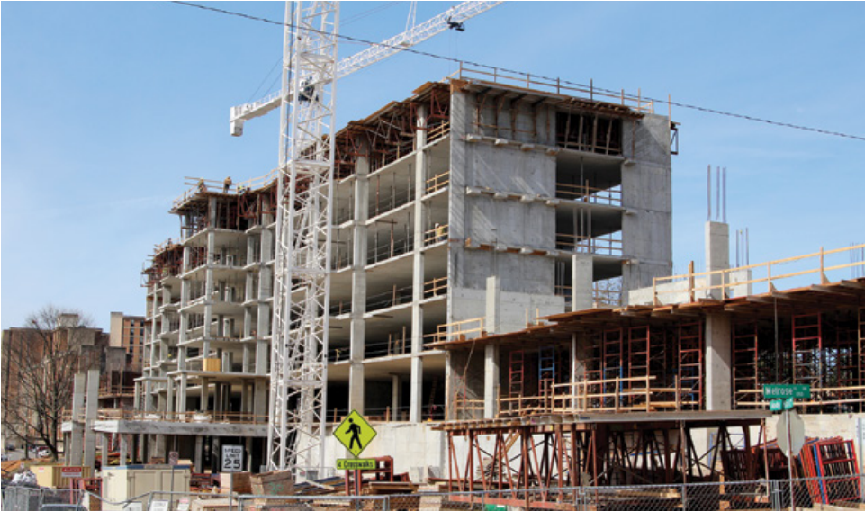
The Health and Information Technology and Simulation (HITS) Laboratory building site.
