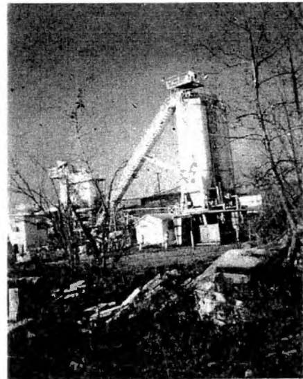
figure 58-An asphalt plant at the southwest corner of the site. Marble pieces from past production at the Marbleworks can be seen in the foreground.
