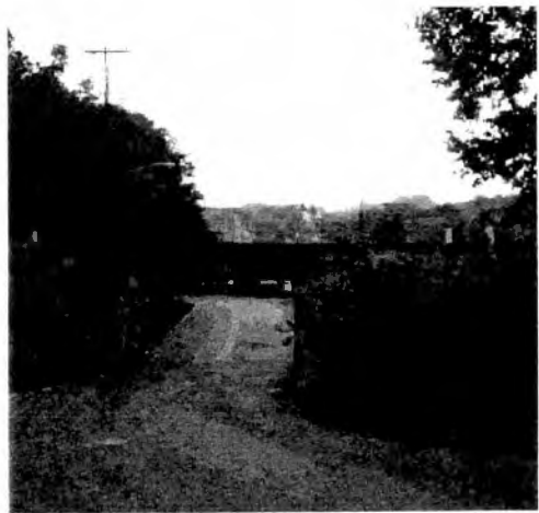
figure 17-Low railroad bridge at a major thoroughfare in Vestal, Tennessee.
