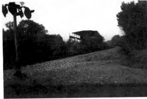
figure 3-Industrial warehouse building, Vestal, Tennessee
