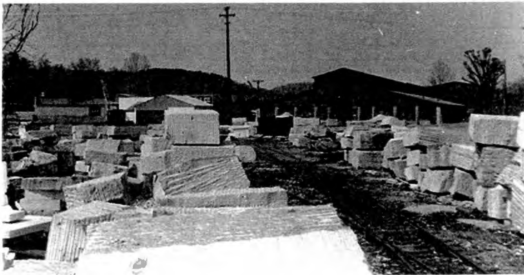
figure 29-View from the marble storage yard to the fabrication buildings, 1947.
