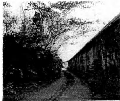
figure 27-Grade change next to the clere-story building, leading to the showroom building at Candoro Marbleworks.
