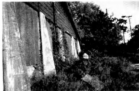
figure 52-The front elevation of the clere-story building, showing the building's twelve foot pilasters.
