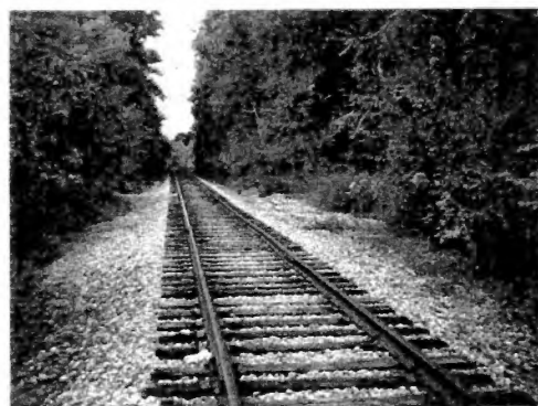
figure 56-L&N railway as it passes the western border of the site.
