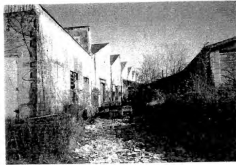
figure 59-View between the sawtooth and clerestory buildings.
