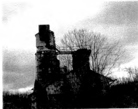
figure 11-Abandoned marble incinerator in Vestal, Tennessee
