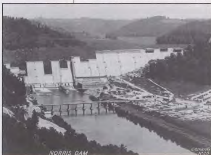
Downstream view of the Norris Dam site in September 1935. Construction of the powerhouse has just started and three overhanging portions indicate the finished height of the dam. Note the cleared valley in the background with the trees representing the future shoreline. (George Palo Collection.)
