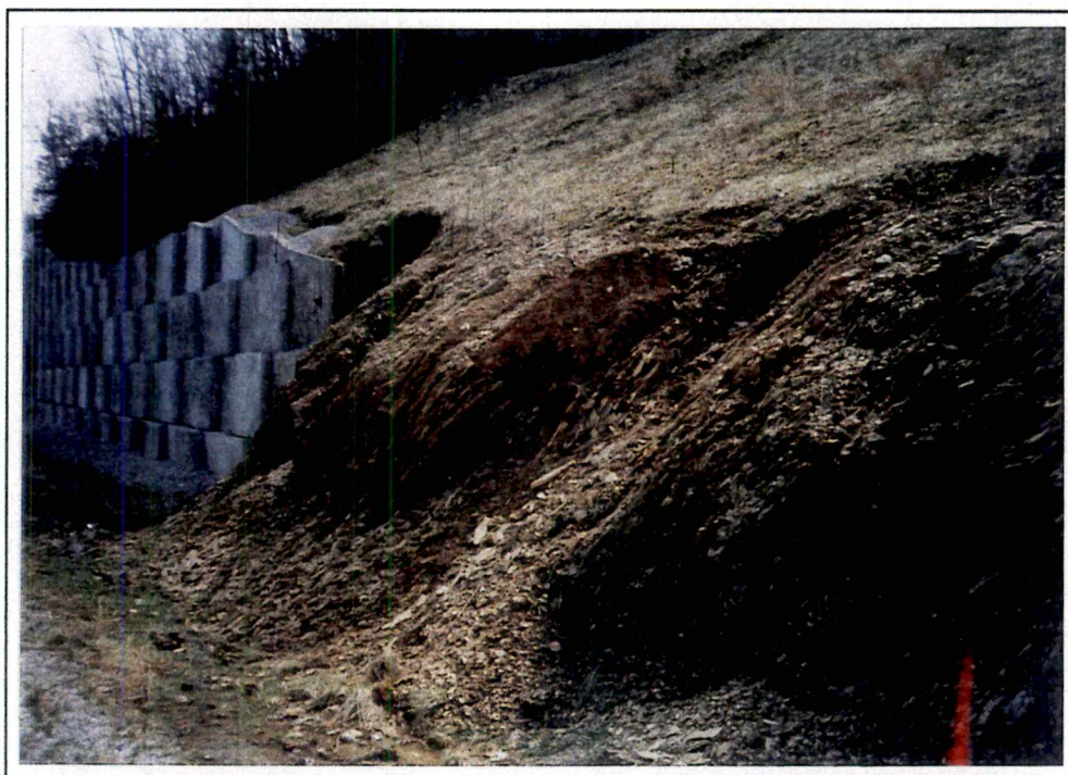
A-1.c Because of the bad weathering conditions in the area a retaining wall was built east of the slope cut.
