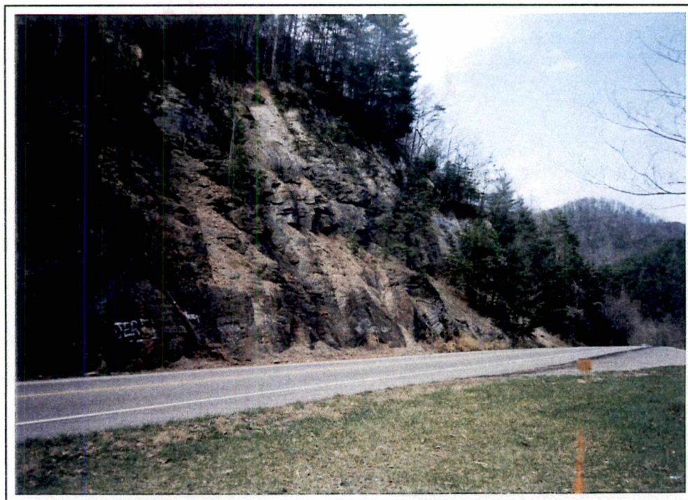
A-5.a General view of the slope showing a moderate degree of weathering.
