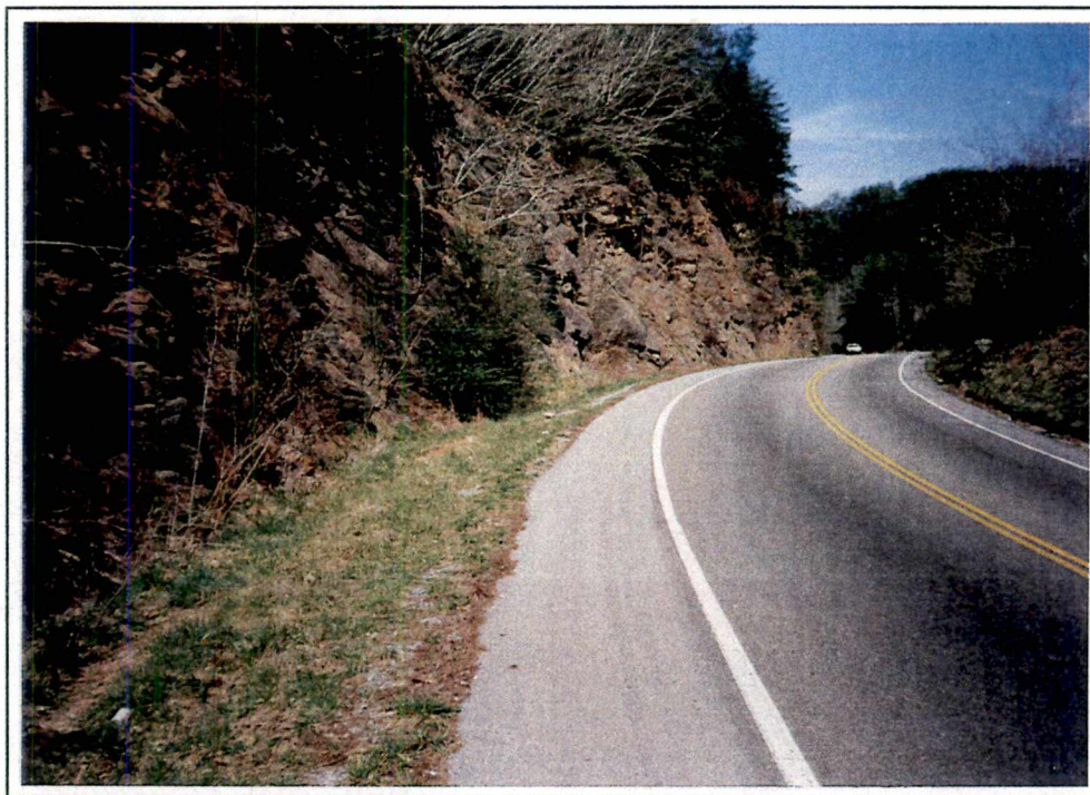
A-2.a Lateral view of the slope rock.
