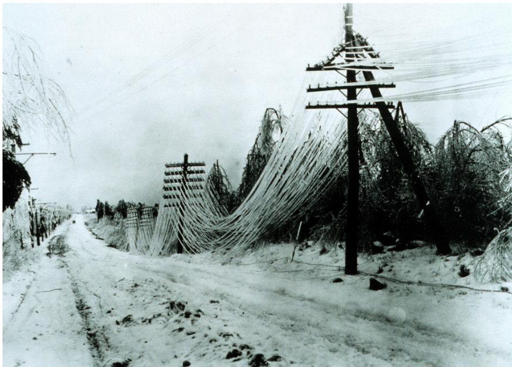
Figure 16: Power Lines During Ice Storm (Source: National Oceanic and Atmospheric Administration)
