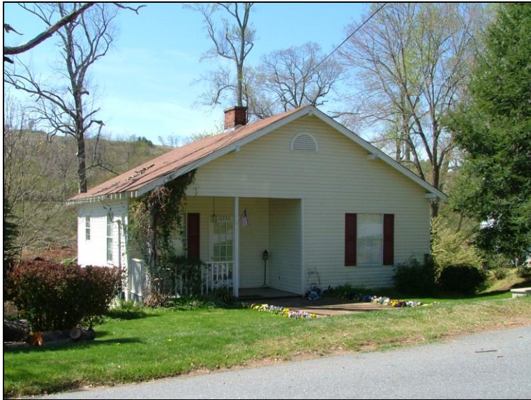
Figure 4.3 Front gabled cottage, Fingerville, Spartanburg County, SC, 2004
