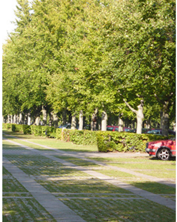
Figure 2.6. Permeable Parking. Source: Build A Better Burb
