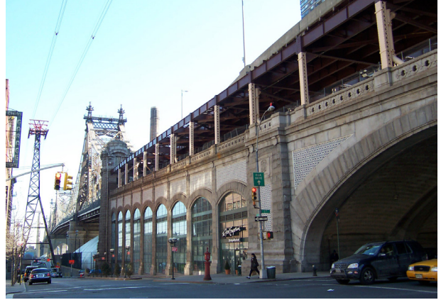
Figure 3.12. Exterior View of Bridge. Source: Michael Minn
