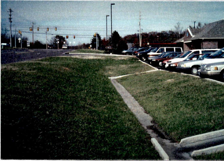
A6.1c - A view looking upstream at the second pond of Pond 6. The dam of this first pond is 2.2 ft. lower than the dam of the second pond and 1.3 ft. lower than the emergency spillway. This pond will overtop before the emergency spillway is utilized. The routed design storm overtops the dam.
