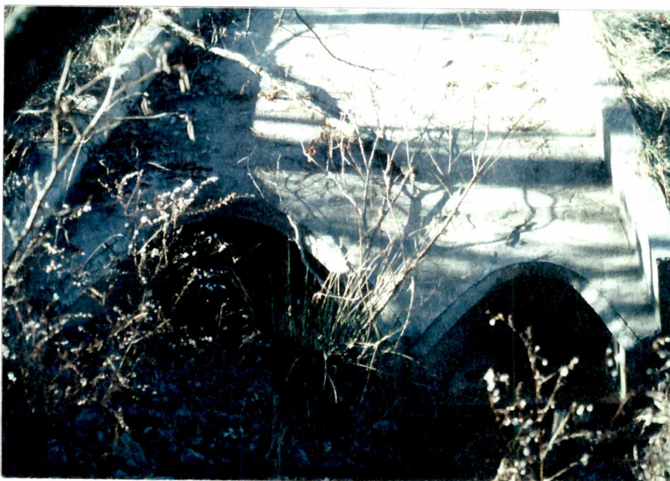
A12.1b - The downstream side of the emergency spillway. The 18-in. diameter pipe on the right is the discharge from Pond 12 and the 30-in. diameter pipe on the left is discharging from the upstream development.
