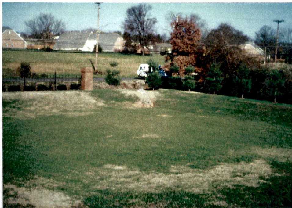
A9.1d - This is an overall view looking downstream at Pond 9. The dam and emergency spillway are in the center of the photograph.
