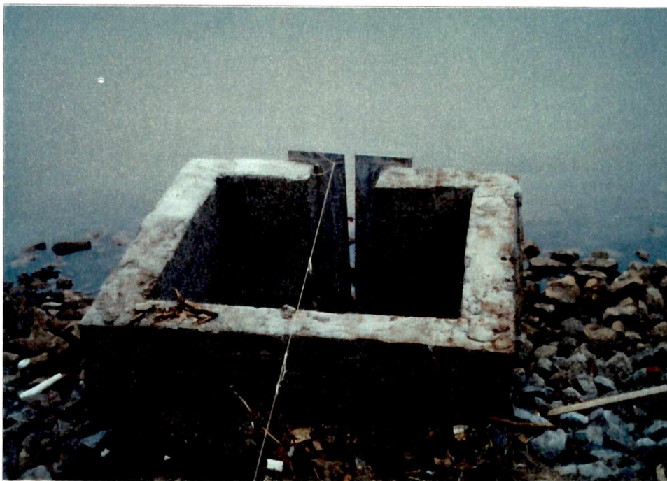
A14.1a - The outlet structure for Pond 14 is a 5 ft. x 5 ft. concrete box having a triangular weir (2.5° notch) outlet control. The invert of the weir is higher than the bottom of the pond so, water always remains in the pond, thus reducing storage space.
