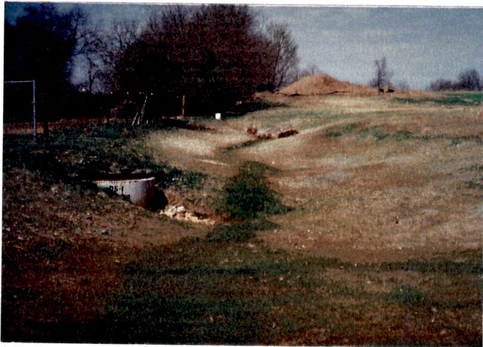
A16.1b - The pond is built to the design drawing plan, but the storage volume at the design depth of 1.3 ft. is only 0.03 ac.-ft., and the design calculations require 0.12 ac.-ft. at the design depth. The design drawing plan does not support the design calculations. The net result is the pond is discharging 1.7 times more than intended during the design storm.
