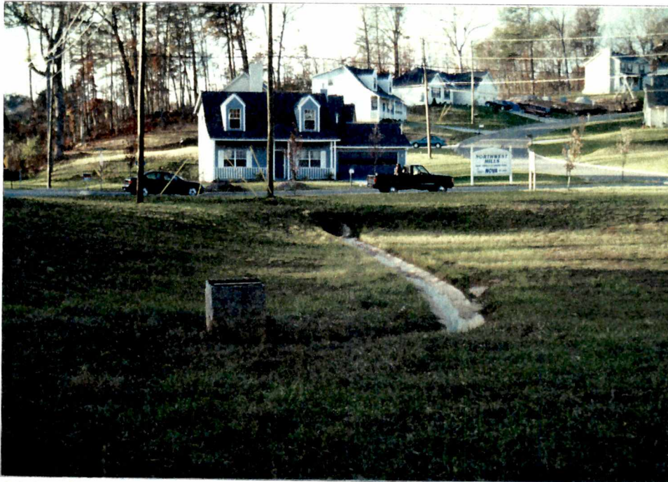
A4.1a - The outlet structure for Pond 4 is a 3-ft. x 2-ft. concrete box having a 12-in. diameter CMP at the bottom of the box for the initial outlet. The initial outlet was intended to be a 4-in. diameter orifice.
