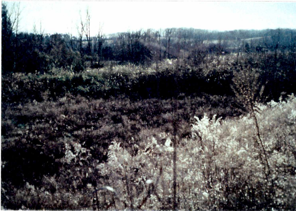
A13.1b - This is a view of the overall pond. The outlet structure is in the center of the photograph in the shaded area. The pond is grown up with weeds and brush and it appears that it is not maintained on a regular basis. The storage volume at the design depth is only 27% of the intended storage volume.
