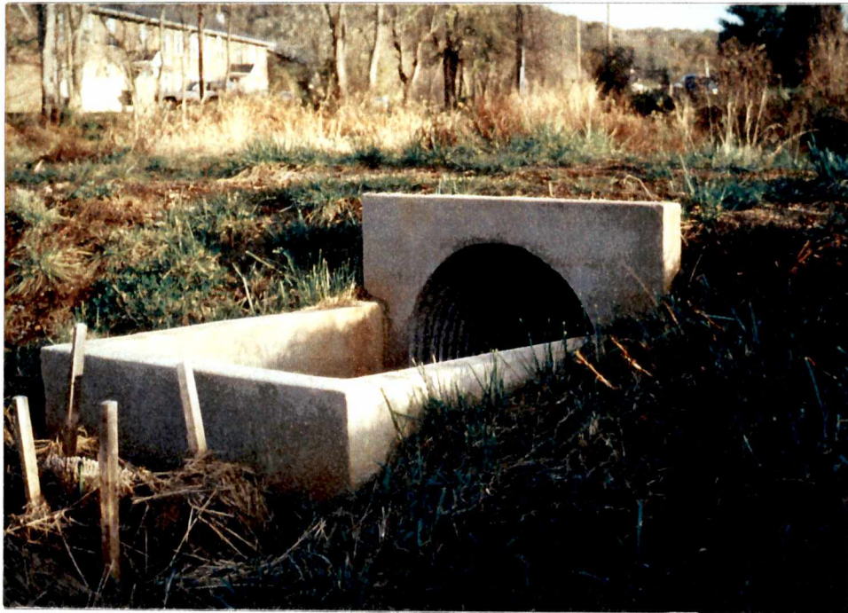
A2.1a - Looking downstream at the outlet structure and dam of Pond 2. The outlet structure is a 5 ft. x 5.5 ft. concrete box with a 12 in. diameter orifice. The orifice is constructed from an 8-in. Diameter PVC pipe.
