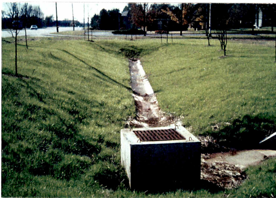
A7.1b - Looking upstream of Pond 7. The sideslopes have a new stand of grass and the bottom of the pond has a 3-ft. wide concrete swale along the length of the pond.
