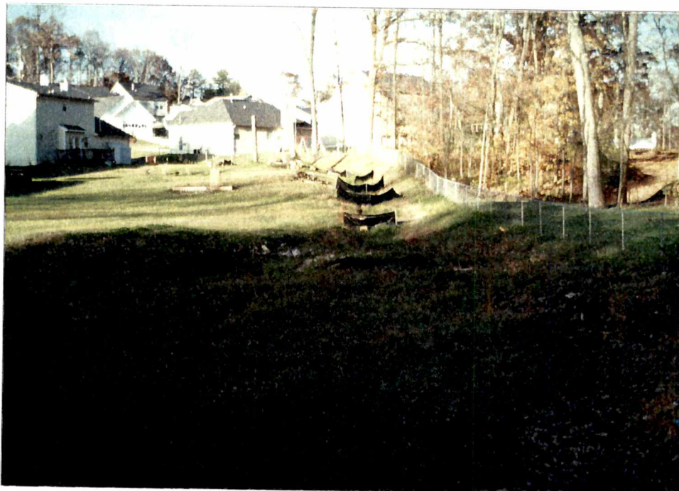
A4.1b - Looking upstream of Pond 4 is an inlet ditch with silt fence erosion protection and check dams. The pond is well maintained.
