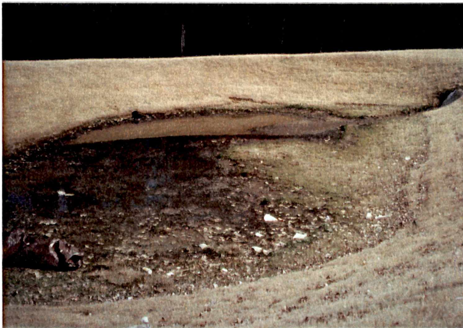
A20.1b - The pond is receiving oil and debris from an upstream parking lot.
