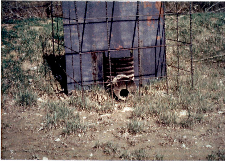
A18.1a - The outlet structure is an 18-in. riser having a 6-in. diameter orifice face plate on the upstream end, an anti-vortex device, and a trash rack.
