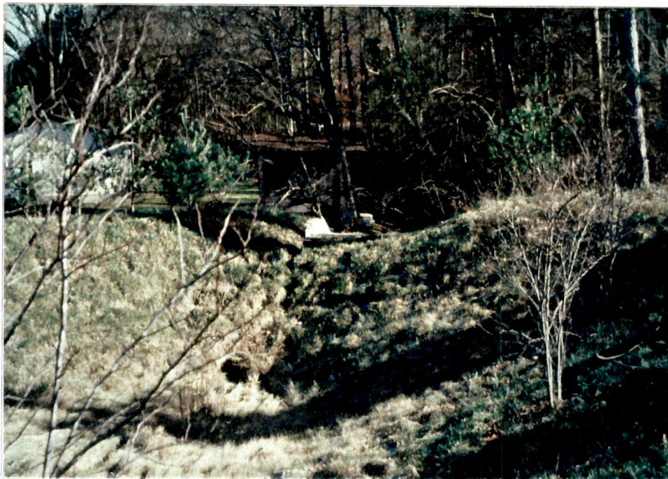
A12.1a - This photograph shows the dam, the outlet pipe, and the concrete emergency spillway. The storage volume in the pond is larger than designed, and is discharging less than the pre-development peak flow. The pond is over constructed.
