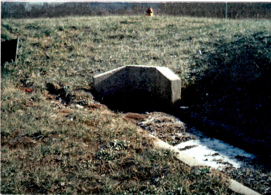
A11.1d - The outlet from the second was designed as an 18-in. diameter RCP having a 13-in. diameter orifice restrictor face plate. The photograph shows that the orifice plate was not constructed. The intended design called for a 5 ft. long x 2 ft. deep grass emergency spillway. The emergency spillway was not constructed.
