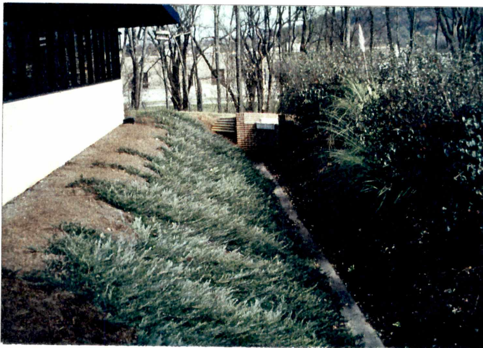
A6.1b - The storage volume for Pond 6 is divided into two ponds. This a view looking downstream of the second pond at the outlet structure. Both ponds are landscaped and very well maintained.
