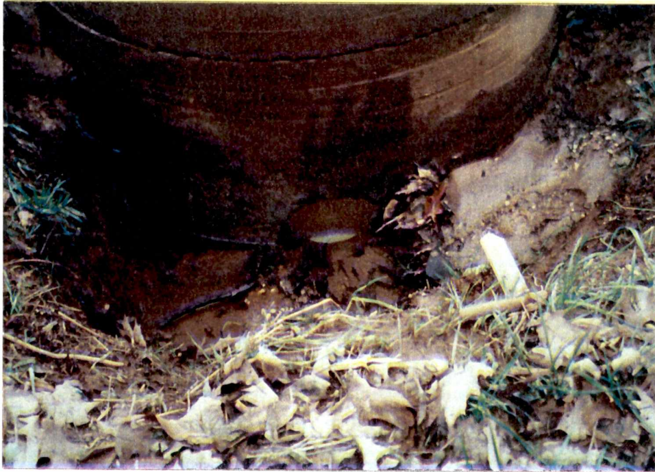
A15.1a - The outlet structure for Pond 15 is a 5-ft. diameter manhole 4.7 ft. high and having a 11-in. diameter orifice at the bottom of the structure.
