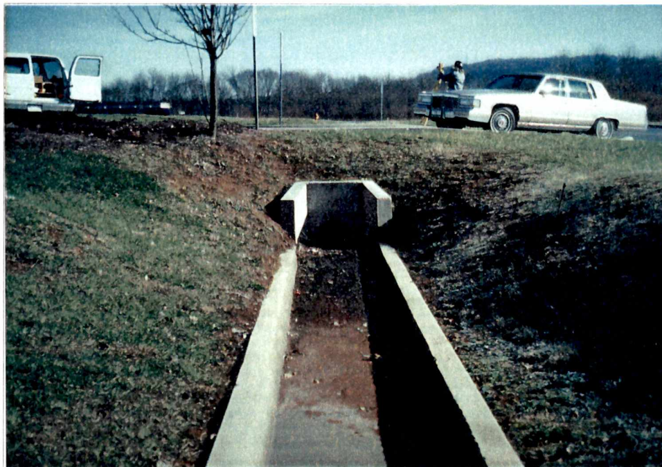
A11.1b - The water is conveyed through an 18-in. diameter RCP from the first pond to the second pond. This photograph shows the inlet end of the 18-in. diameter RCP.
