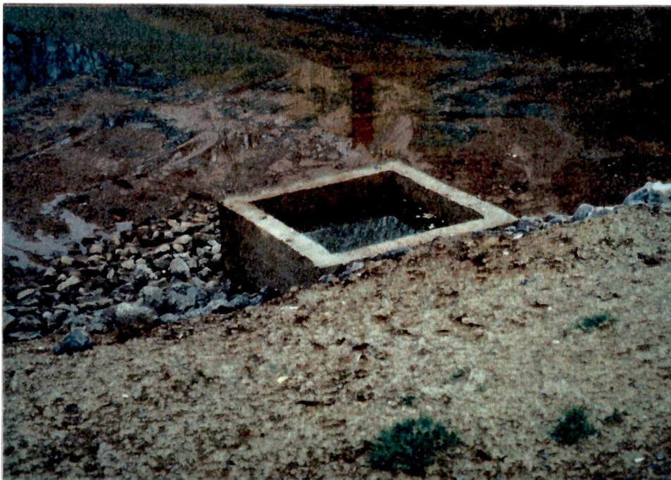
A14.1d - The inlet to the pond is a 5 ft. x 5 ft. concrete block box with a 48-in. diameter inlet pipe. The box does not have an outlet at the bottom therefore, the box stays full of water until it evaporates. The actual storage at the top of the dam is 52% of the intended storage volume. The actual measured dam height is 2.9 ft. lower than designed. The dam overtops during the design storm.
