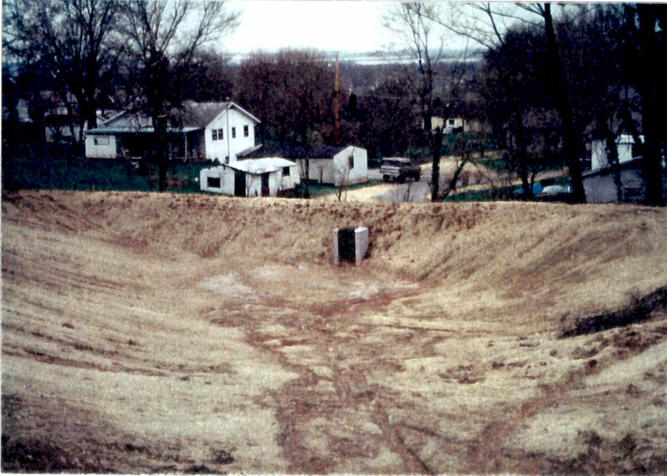
A17.1b - The actual storage volume at any given depth is less than the storage volume as represented by the design plan drawing and shown in the the design calculations. The design plan drawing storage volume at any given depth is less than the storage volume shown in the design calculations. The net result of inadequate storage is that the pre-development peak flow is being exceeded for the design storm.
