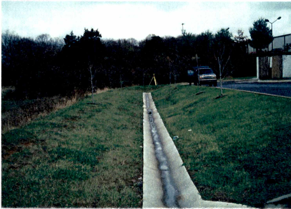
A8.1c - This is a view looking downstream at the dam (left side of the photograph). The downstream resident complains of excess water being discharged onto his property.
