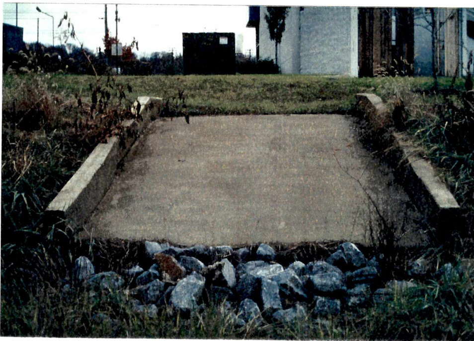
A8.1b - This is a view of the emergency spillway looking upstream. The spillway is 9 ft. long and 11 inches deep and the design specified a length of 9.6 ft. and a depth of 11 inches.
