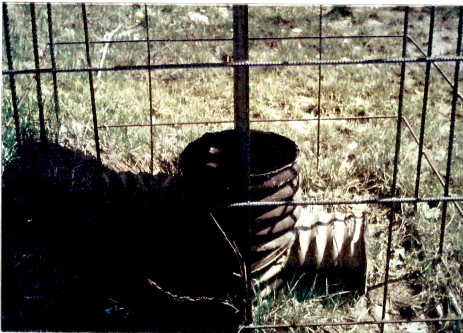
A18.1b - The side view of the outlet structure.
