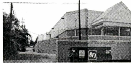
Fig. 6.19 The view along the alley behind Walgreens. The massive retainer walls will pose a challenge to planning service circulation and parking.
