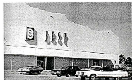
Fig. 4.28 Best store. The building is a big box with windows located only at the entrance. Source: Rowe.
