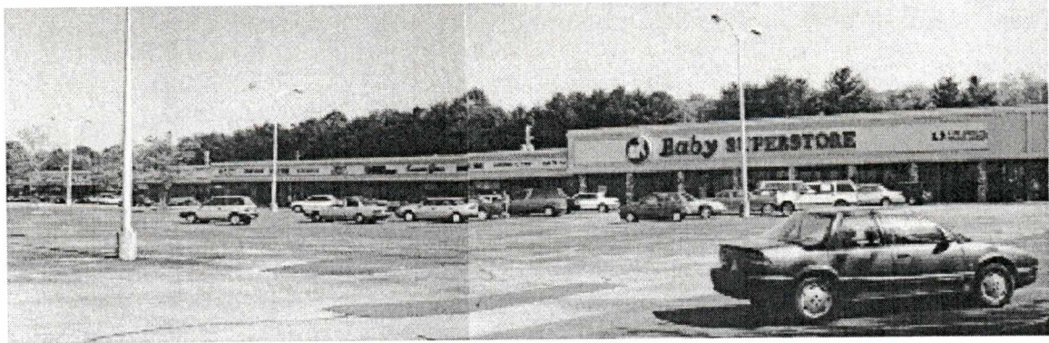
Fig. 4.2 Suburban retail strip development. Cedar Bluff Shopping Center in Knoxville, Tennessee, 1995.
