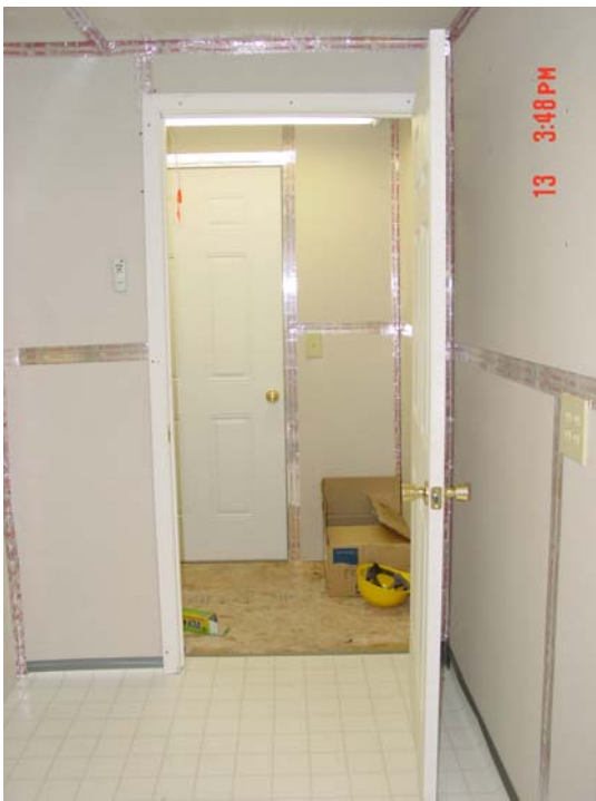
Figure 13. Photograph from inside main room of indoor structure. Front door and foyer are visible through open second door.
