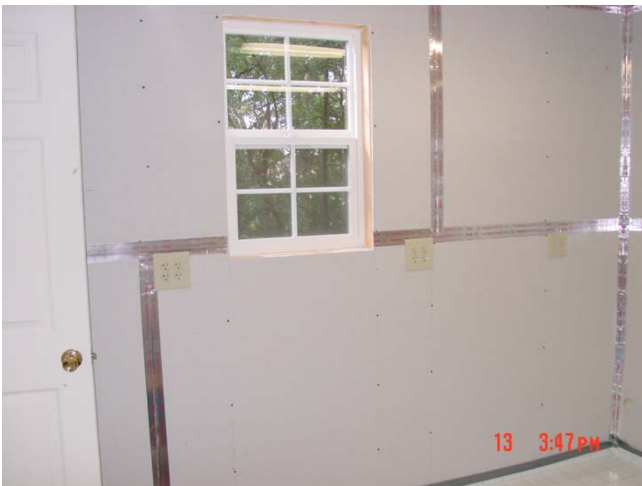
Figure 15. Photograph of west wall of main room showing second window in main room and multiple electrical sockets.
