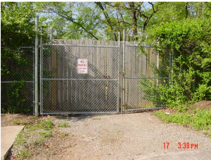
Figure 9. Front gate of ARF showing wooden and chain-link fences.
