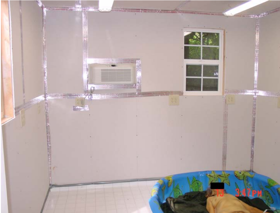
Figure 14. Photograph of north wall of main room showing air conditioner and window. Thermometer eventually placed next to window shown.
