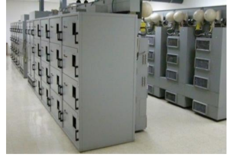
(b). Transmitter station
