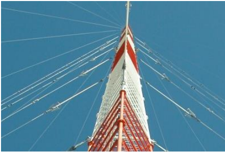
(c). Transmitter tower
