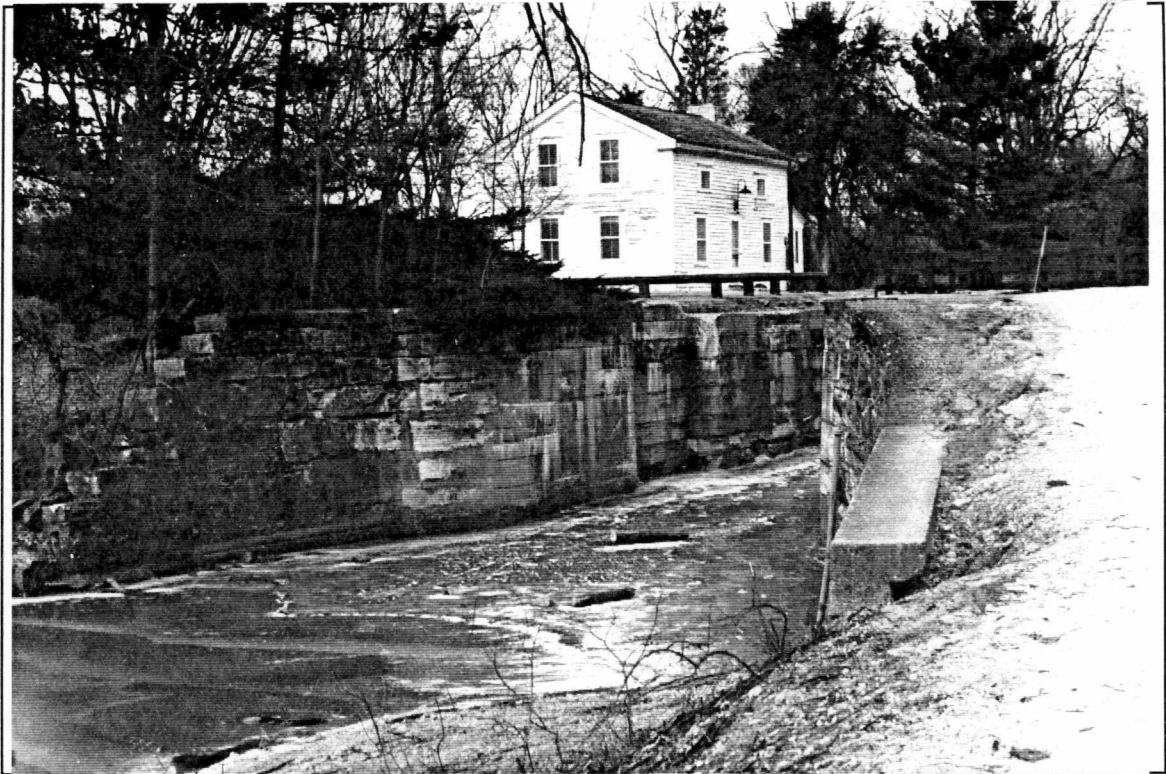
Figure 4-5. Lock 6 and Locktender's House.
