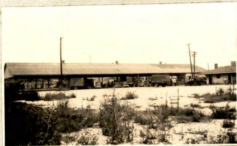
Chattanooga Wholesale Truckers Shed, 200 feet in length. Rear space in foreground for future expansion (3 1/2 acres total market area). Restaurant and office on right.
