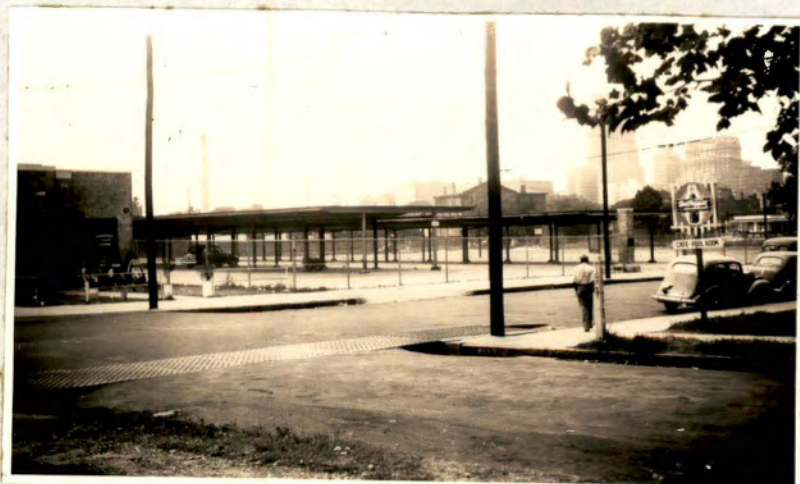
Three acres space; 2 sheds; restaurant, office, seed store, packing rooms and garage on left.
