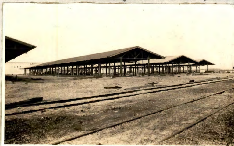
Figure 50. Kansas City Food Terminal (under construction, Sept. 4, 1939).
