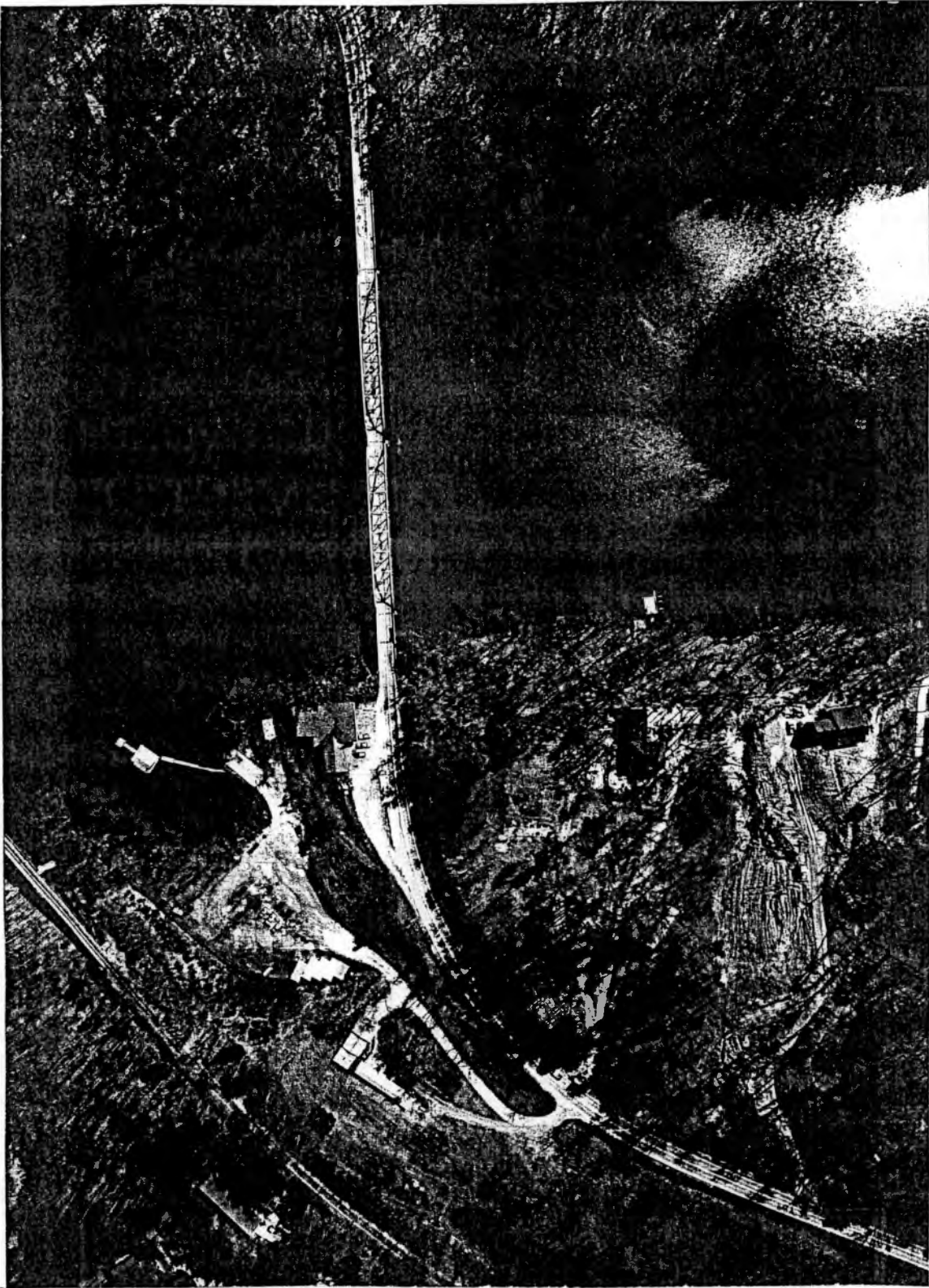
Figure 9: An aerial view of existing bridge
