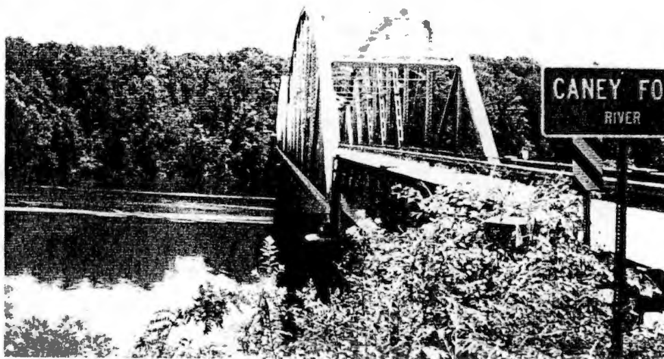
Figure 7: View showing spans 5 and 6, steel trusses
