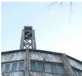
Figure 1.17: Staro Sajmište. Tower Detail (2014).
