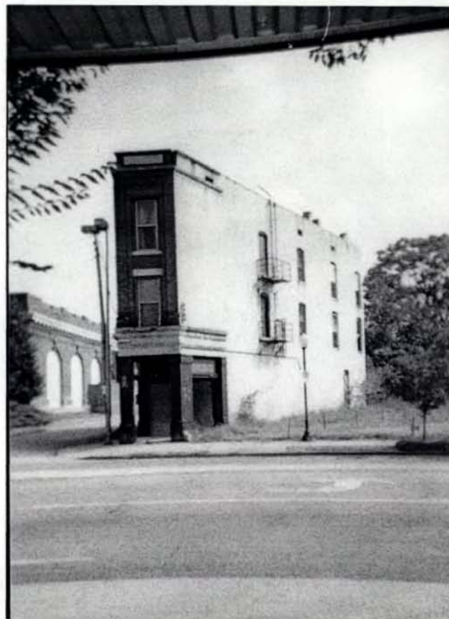
Above: The entry to what was once Rich's in the Strong Building as seen from South Market Street
