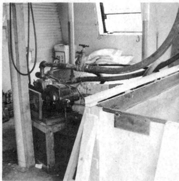
Figure 3. Model tank and pumping equipment.
