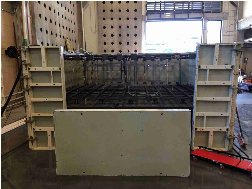
Figure A.6: Partially assembled side formwork system
