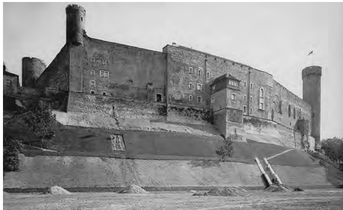
Renovated wall after the construction of the Parliament building.
