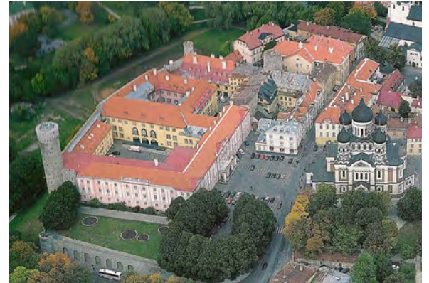
Aerial view of Parliament building as it was built into the foundations of the old Castle walls.
