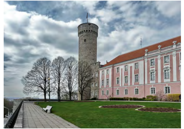
View of the intimate connection between old and new construction.
