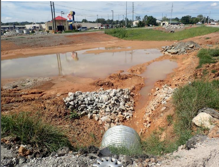
SR-33 and Beaver Creek Road intersection Improvements, Knox Co.
