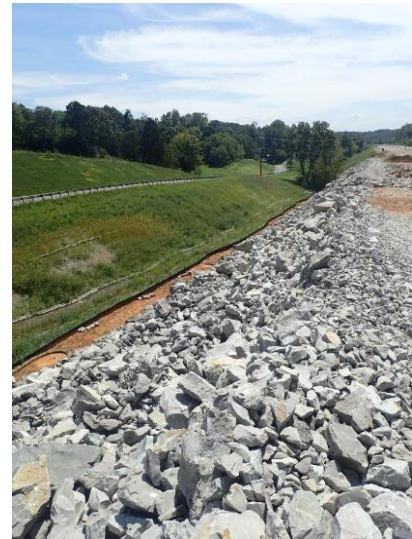
Proposed roadway fill with temporary berm (EC-STR-27). Temporary slope drain has not been installed yet.
