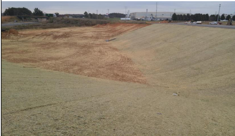
Temporary slope protection (EC-STR-34).
