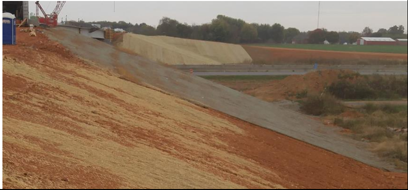
Erosion control blanket used for slope Installation (EC-STR-34)
