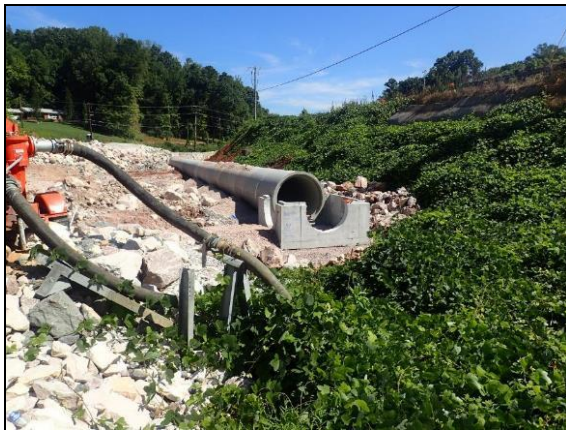
Suspended pipe diversion (EC-STR-33A) Upstream side
