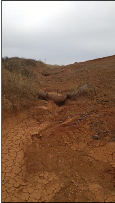
Sediment tube used for ditch application (EC-STR-37)
