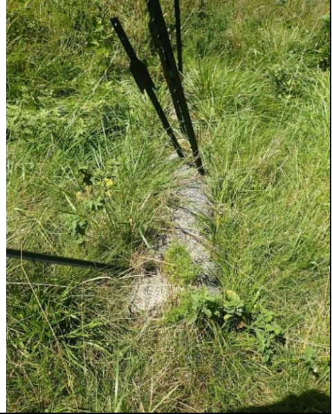
Filter sock (EC-STR-37). Short piece of geo-hay tube staked using steel posts.
