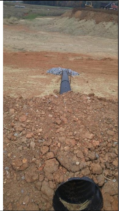
Temporary slope drain (EC-STR-27).
