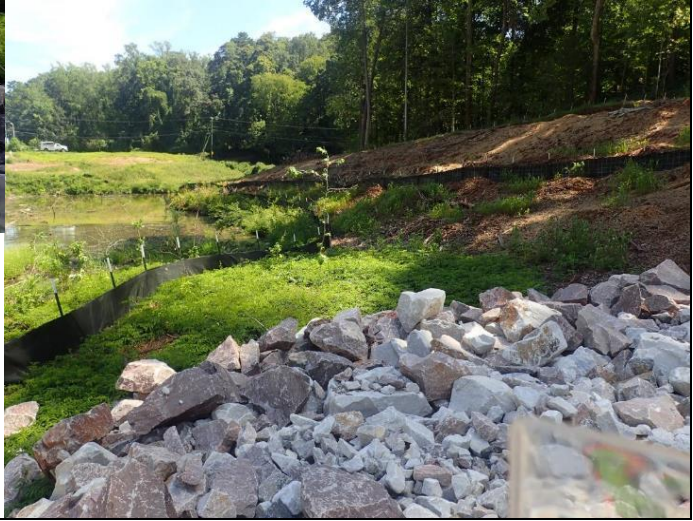
Silt fence with wire backing (EC-STR-3C) used around bodies of water.
