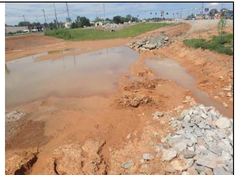
Permanent drainage basin
