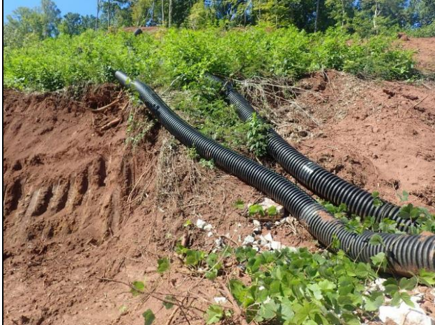
Temporary slope drains (EC-STR-27)
