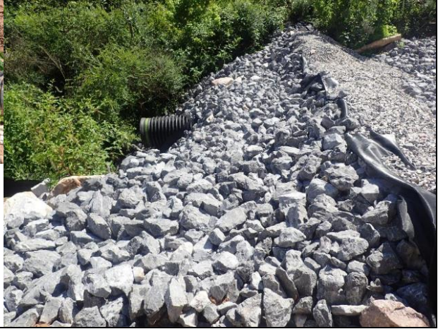
Enhanced rock check dam (EC-STR-6A) shown with temporary slope drain outlet
