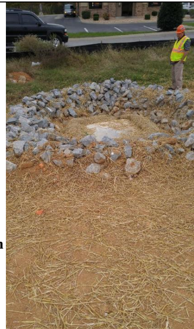
Catch Basin Protection (type B) with sediment tubes (type D) and temporary mulch (EC-STR-19).
