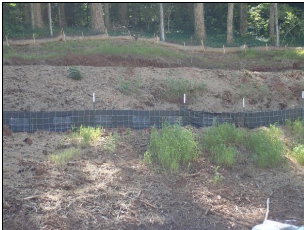
Sediment tube used as a berm (EC-STR-37). Silt fence with Wire Backing used in the middle of cut slope (EC-STR-3C) .
