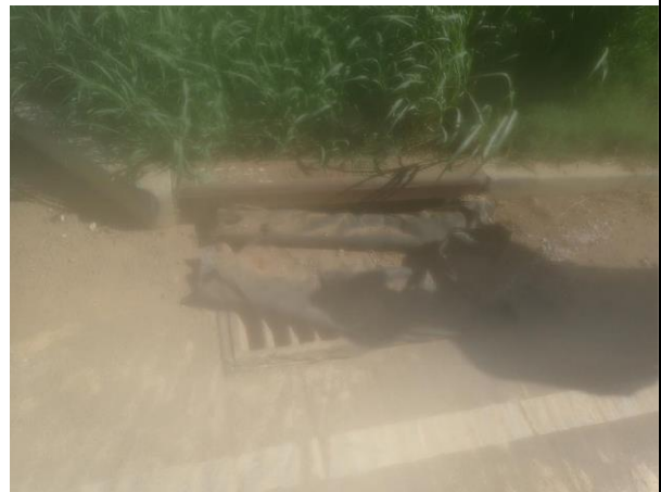
Curb inlet protection, Type 4 (EC-STR-39A)
