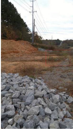
Looking downstream from the proposed lane of the roadway widening project.
