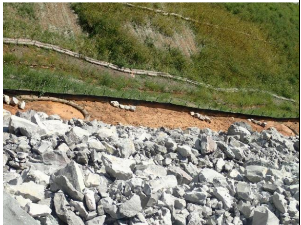
Silt fence with wire backing (EC-STR-3C) used with rock or sediment tube weirs. Two rows of sediment tube used on the other bank.
