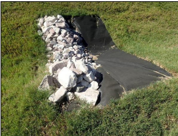
Rock check dam (EC-STR-6)
