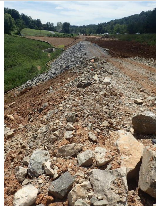
Proposed roadway fill with temporary berm (EC-STR-27). Temporary slope drain has not been installed yet.
