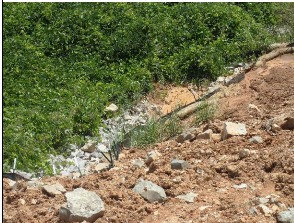
Silt fence with wire backing (EC-STR-3C) used with sediment tube at the toe of fill slope.
