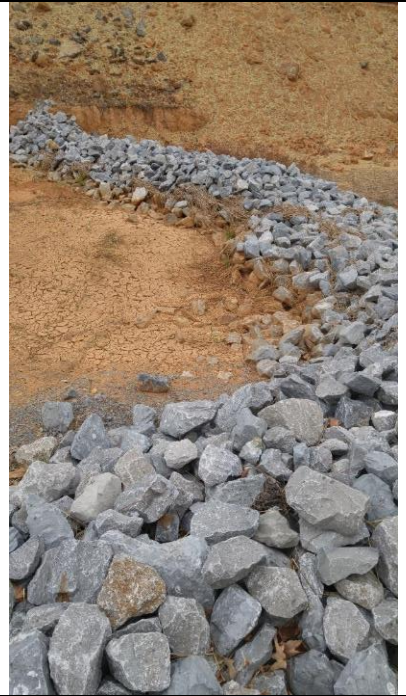
Rock Check Dam (EC-STR-6).
