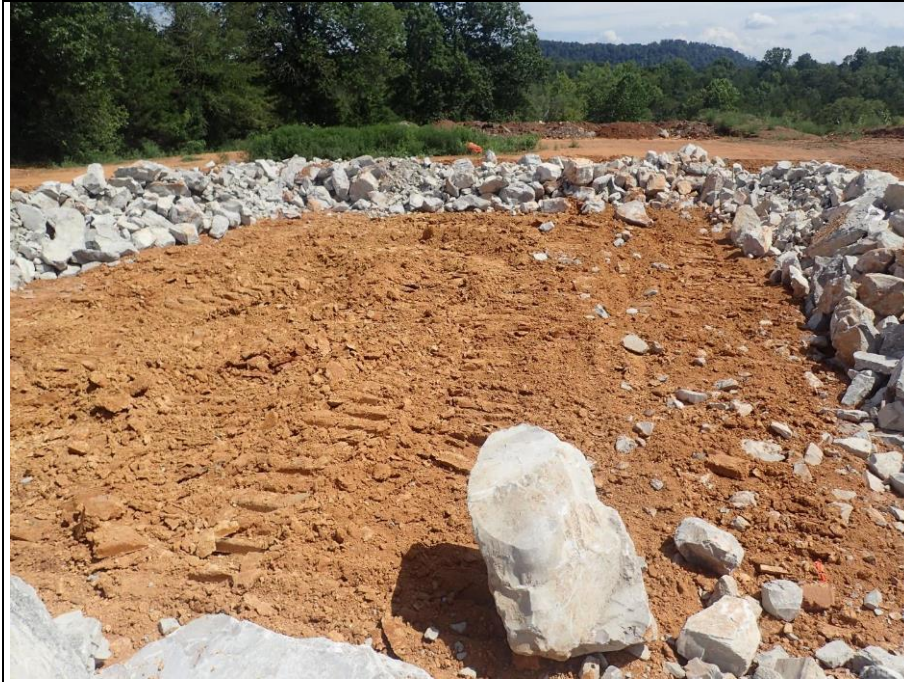
Dewatering structure under construction (EC-STR-1).
