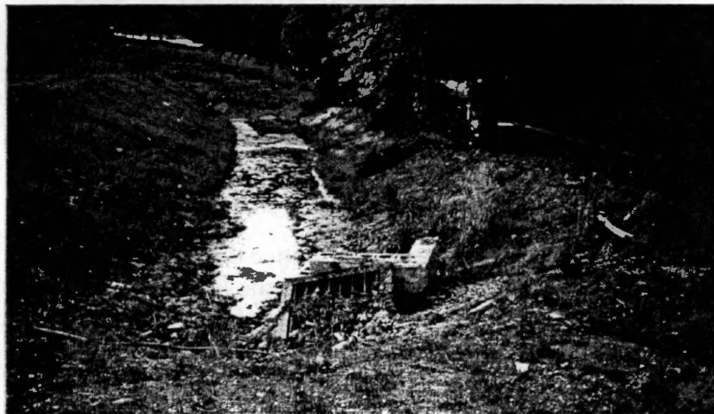
Figure E.2- Longitudinal view of pond. Notice the large amount of trash and debris in and around the pond. The outlet control structure can be seen in the foreground. Standing water would suggest clogging in the outlet control structure, if 48 to 72 hours have passed since the last rainfall. In the distance, notice the erosive action on the inlet channel.
