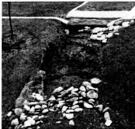
Figure 5.4- View of Inlet from Opposite Side of Pond
