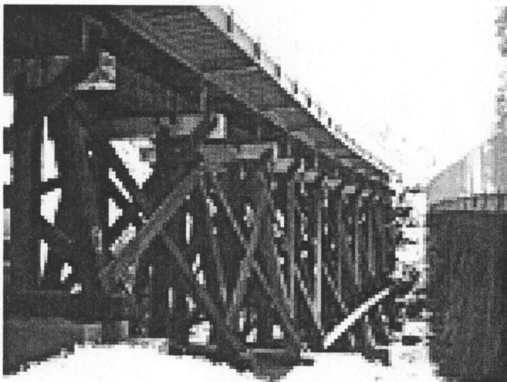
Fig. 1.27: Recycled trusses. The trusses in the railroad bridges found on the site are also being reused. The railroad structure—ties and all—currently support roads which seem to have been used for automobiles at one time but which are now used for pedestrians and cyclists. Source: Author.
