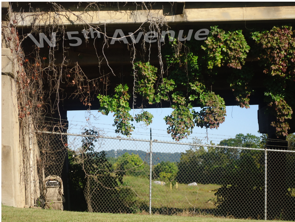
Figure 16. View under West 5th Avenue.
