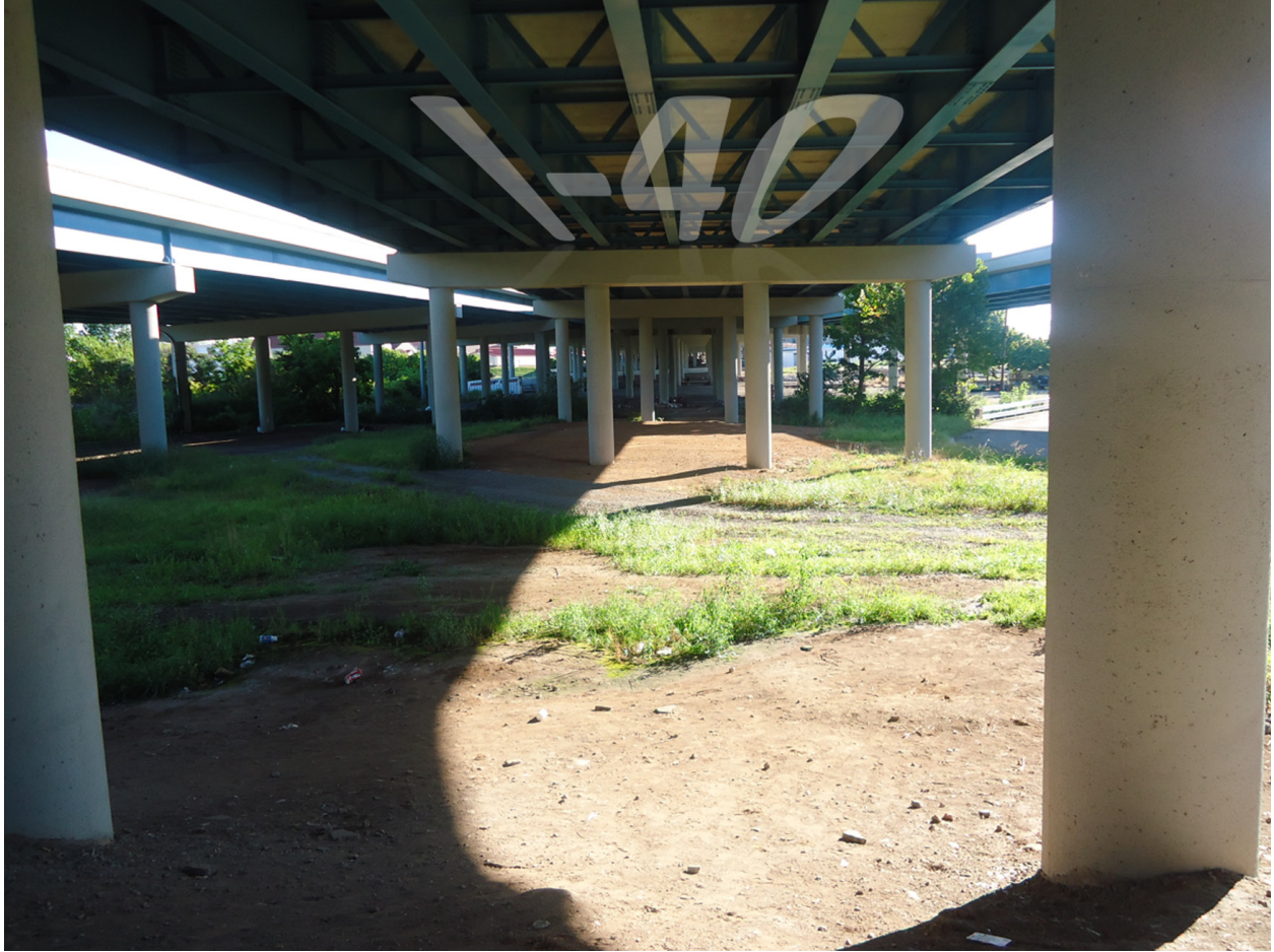
Figure 15. View under Interstate 40 looking east.
