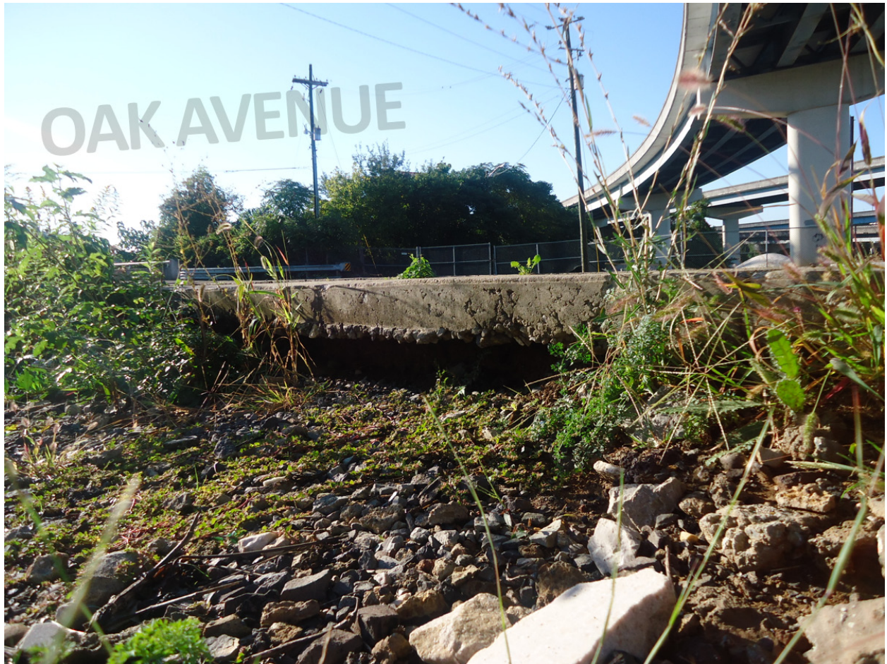
Figure 14. View at Oak Avenue.
