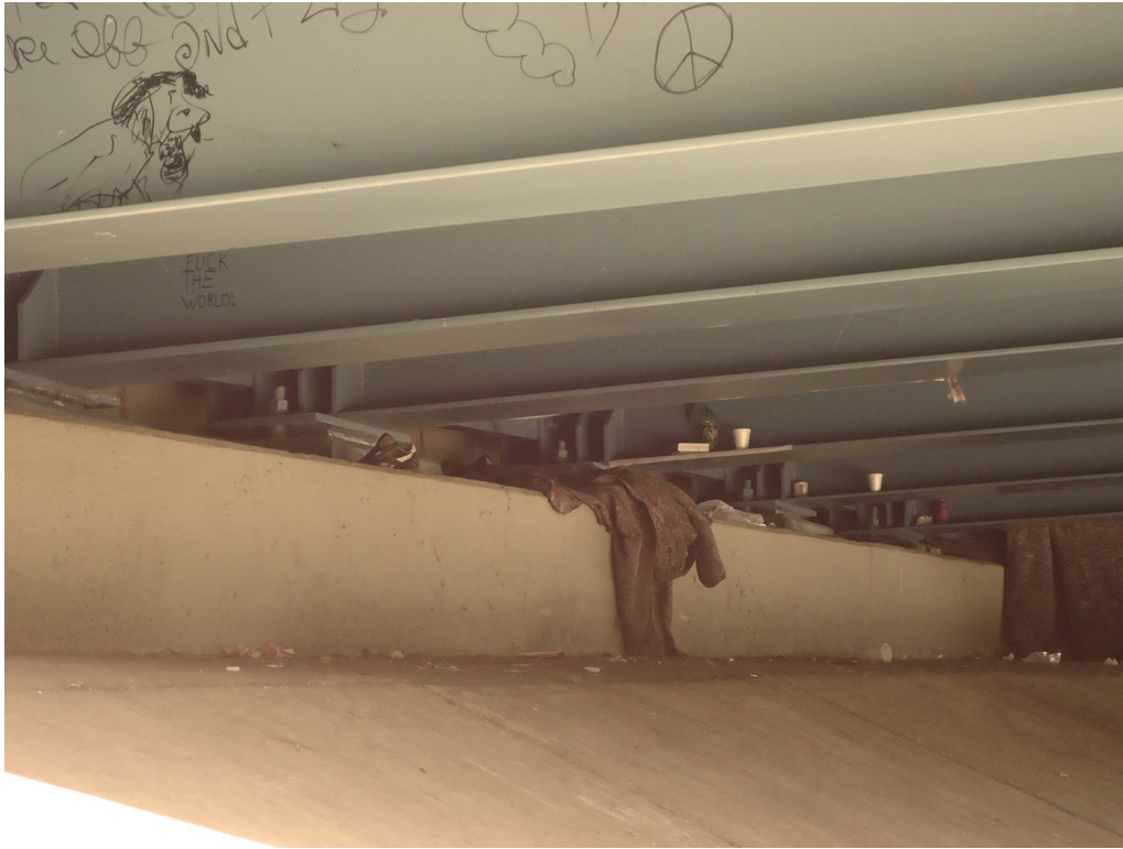
Figure 19. Living space is produced under Interstate 40.
