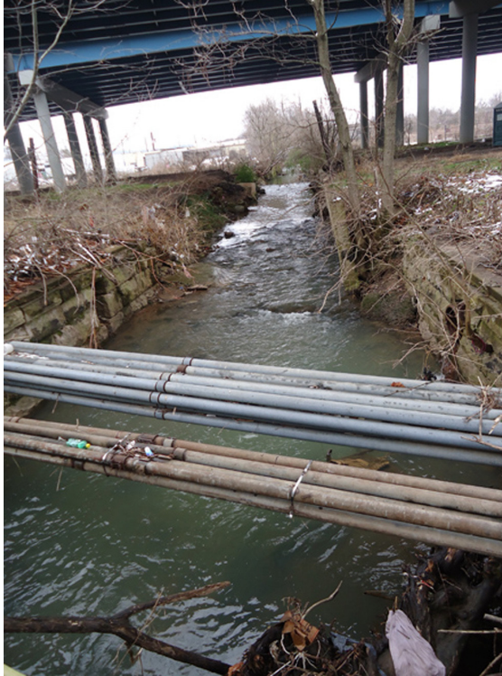
Figure 11. Second Creek under I-40.
