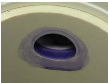
A View from the inside of the pipe of the sharp branch edge.
