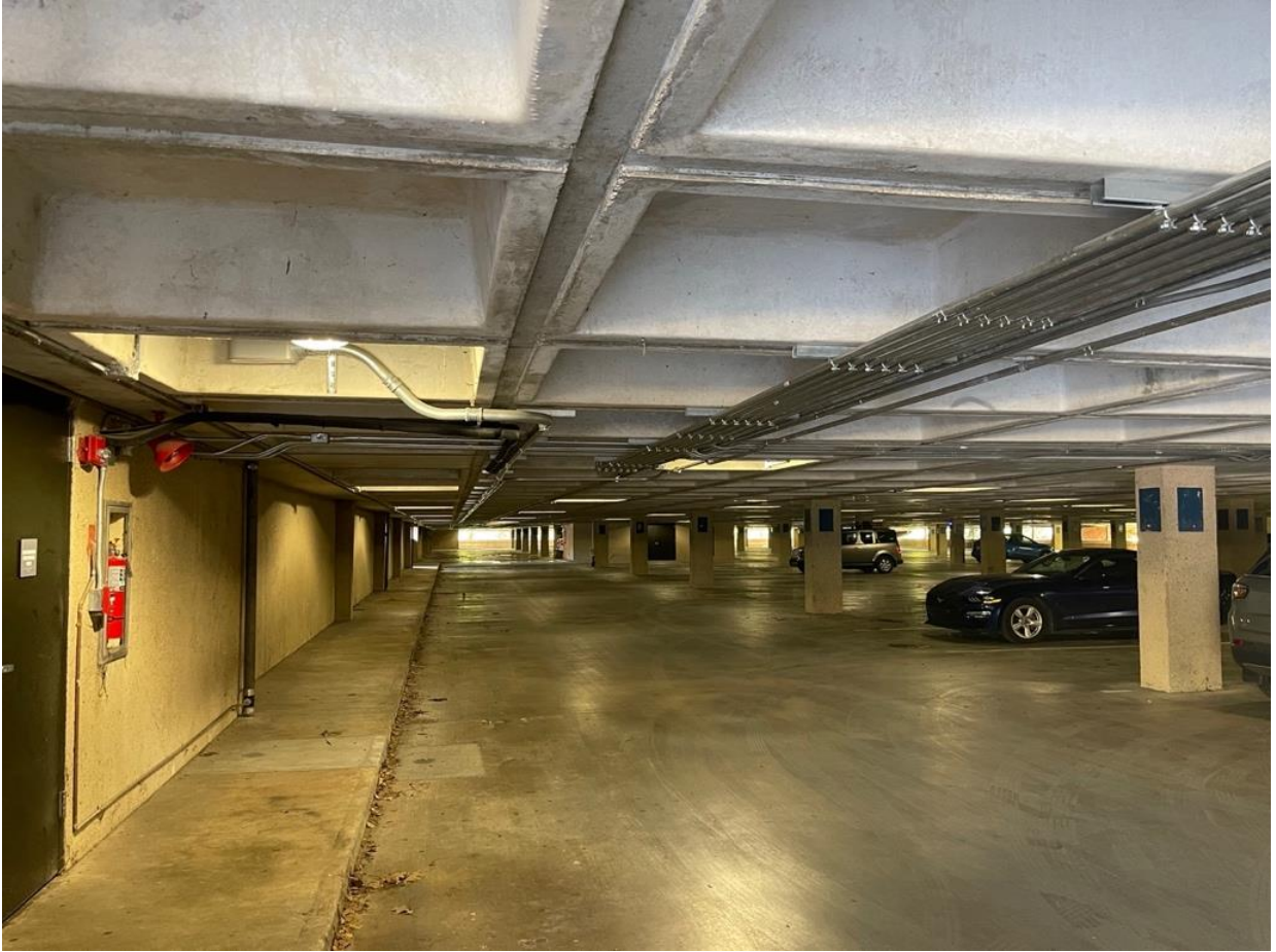
Figure 4.6. Parking garage on Clarissa's campus.
