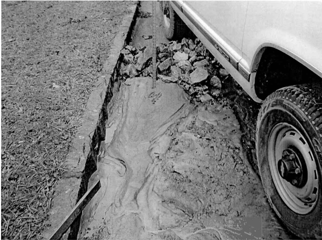
Figure 3-5. Photograph of Chimney Tops check dam with trapped sediment
