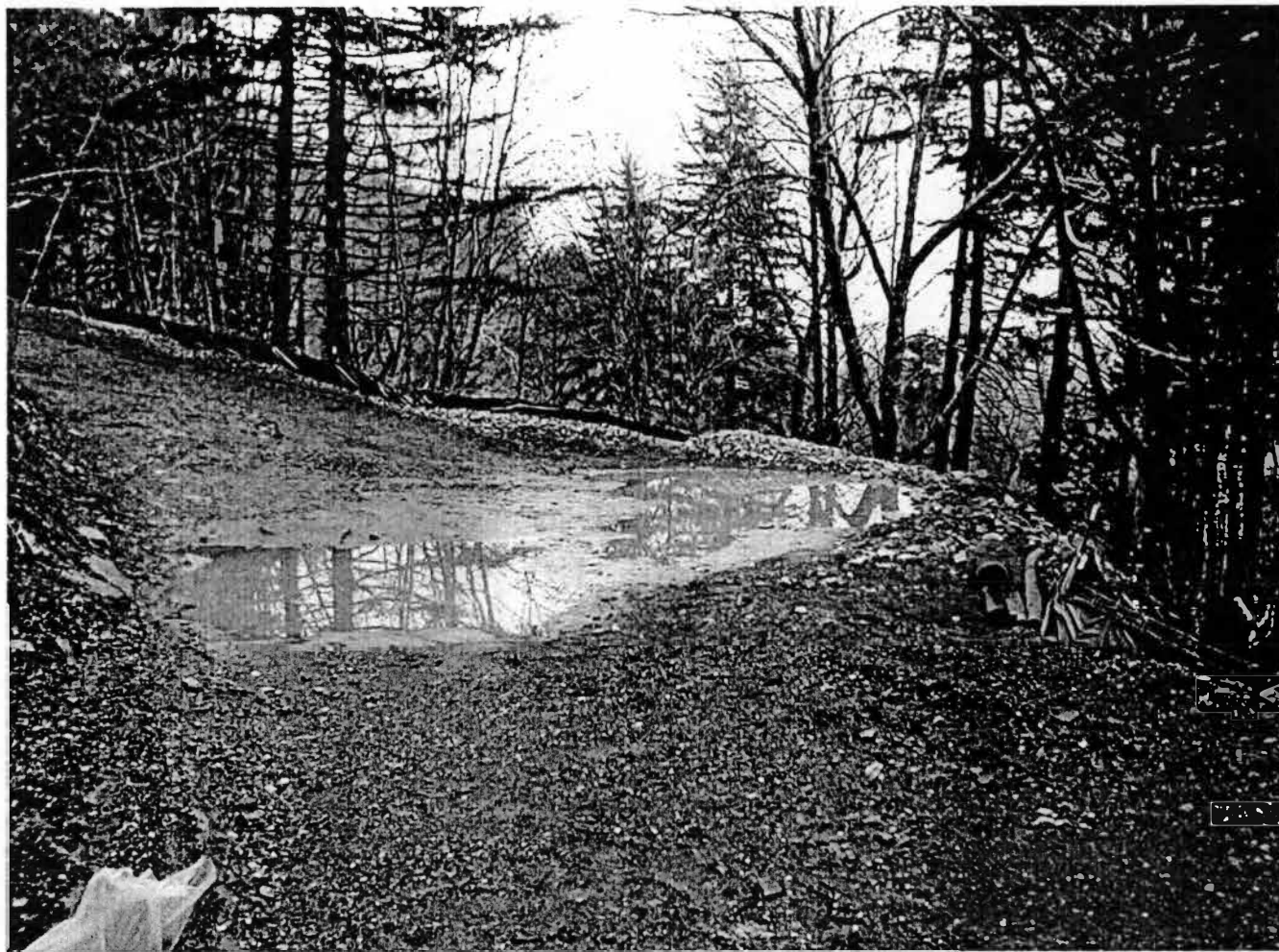
Figure 3-8. Old Trace Road rock check dam
