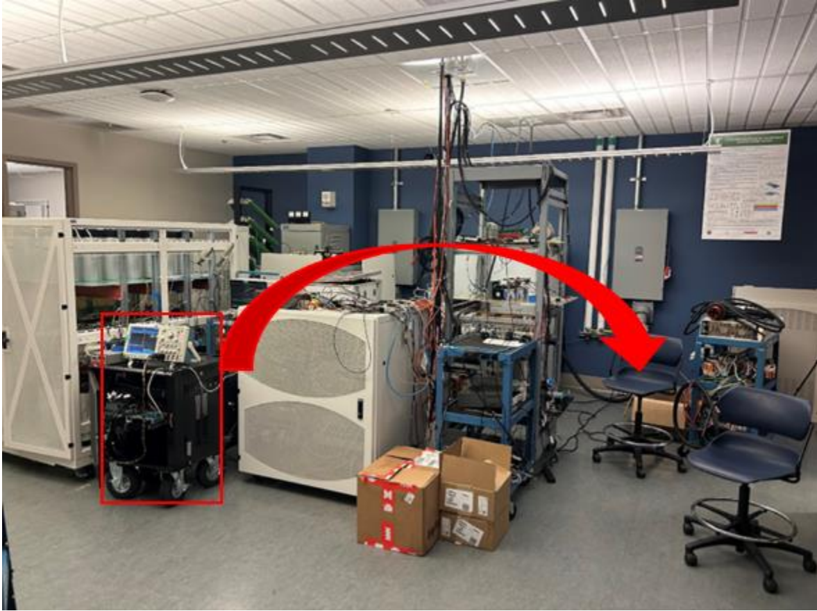
Figure 6.17. The controller moved away from the converter cabinet.
