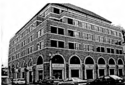
Fig. 48: A facade of a Center Square Building.
