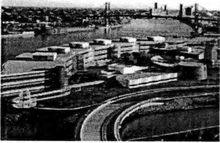
Fig. 33: View of the Owens Corning complex. Source: Russell
