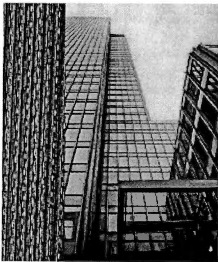
Fig. 10: A facade of the Seagram Building.
